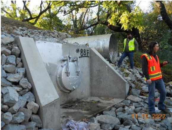
An outfall being rehabilitated
