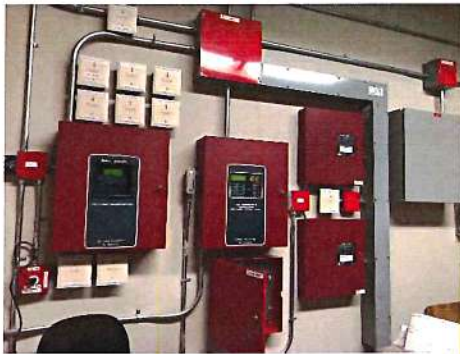
* PAC Fire Alarm System Replacement
