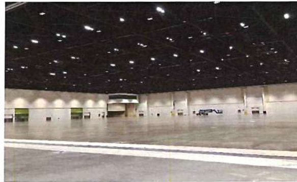
* Convention Center Exhibit Hall Lighting and Ceiling Upgrades
