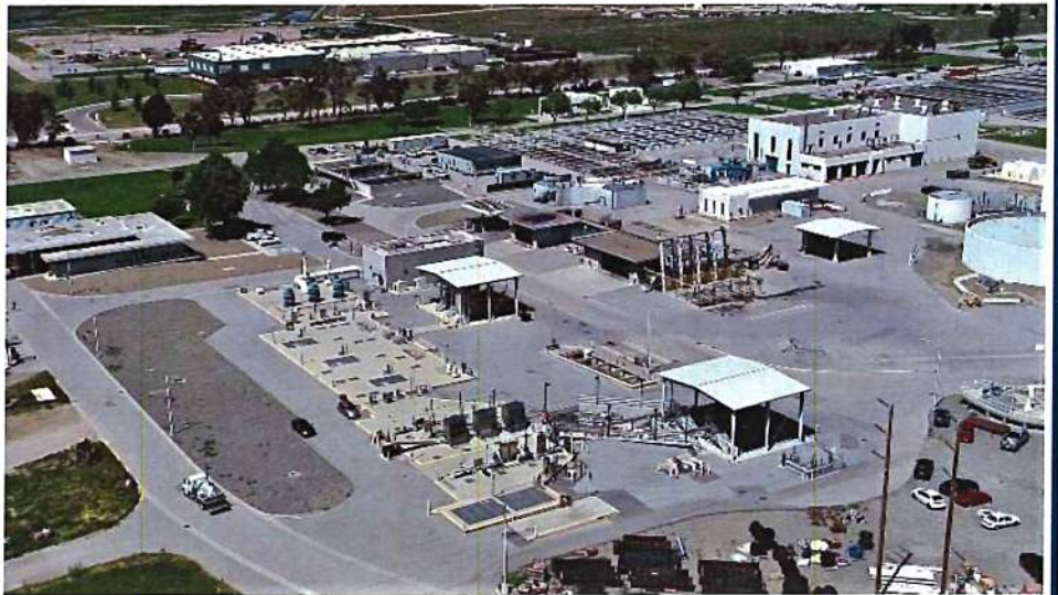
Headworks Critical Improvements
