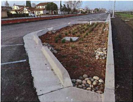
* Chynoweth Avenue Green Street Project
