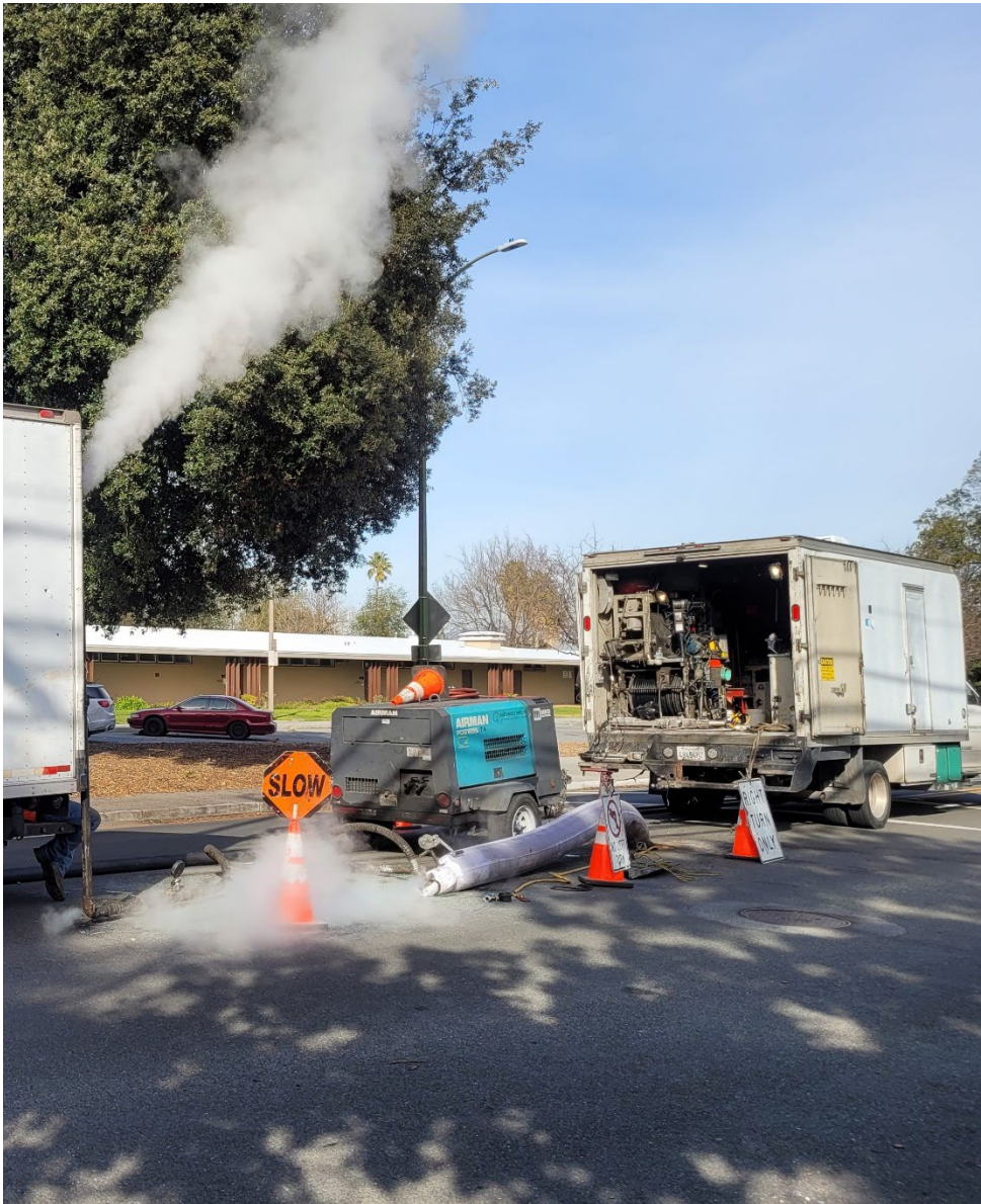
Cast-In-Place-Pipe (CIPP) Liner Installation
