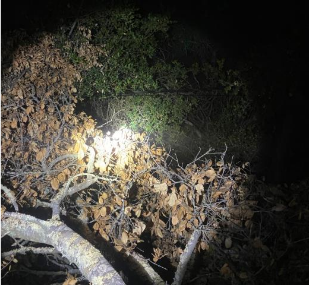
Figure 33: Vegetation-Hazard in Sonoma County – Tree fell on service wire
