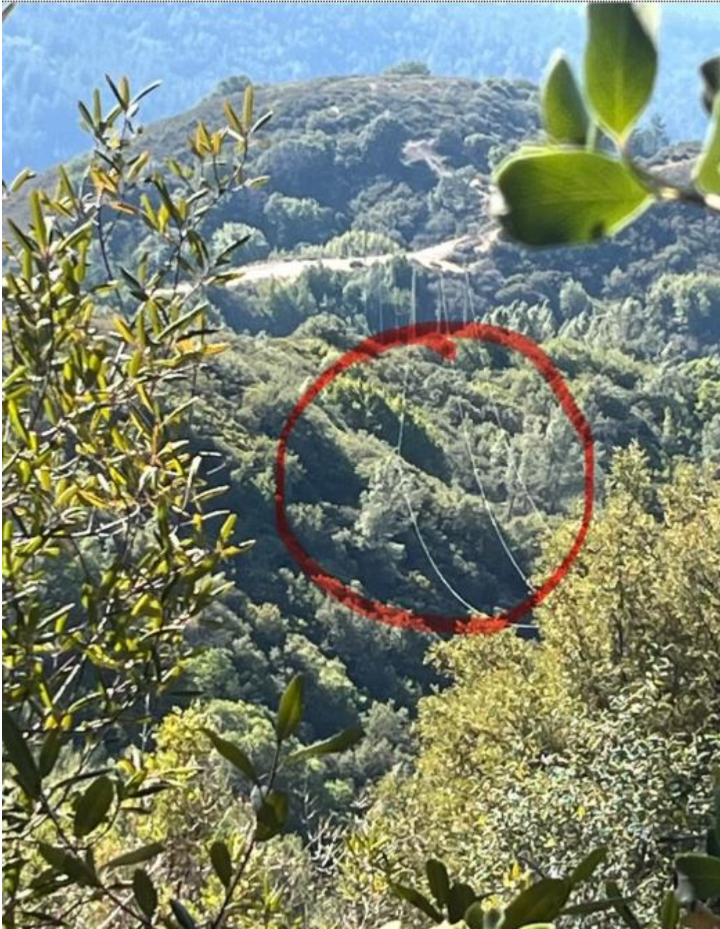
Figure 27: Vegetation-Damage in Santa Clara County – Tree on line
