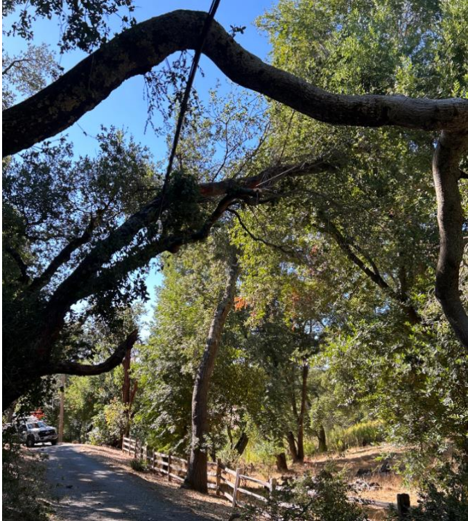
Figure 34: Vegetation-Hazard in Sonoma County – Tree fell on service wire
