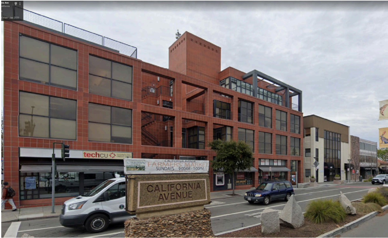
FAIL Palo Alto California Avenue at El Camino. Inadequate design standards.
