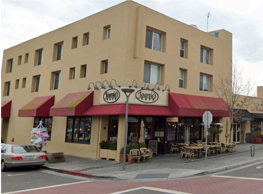
FAIL Palo Alto California Ave at Ash, Inadequate design standards.
