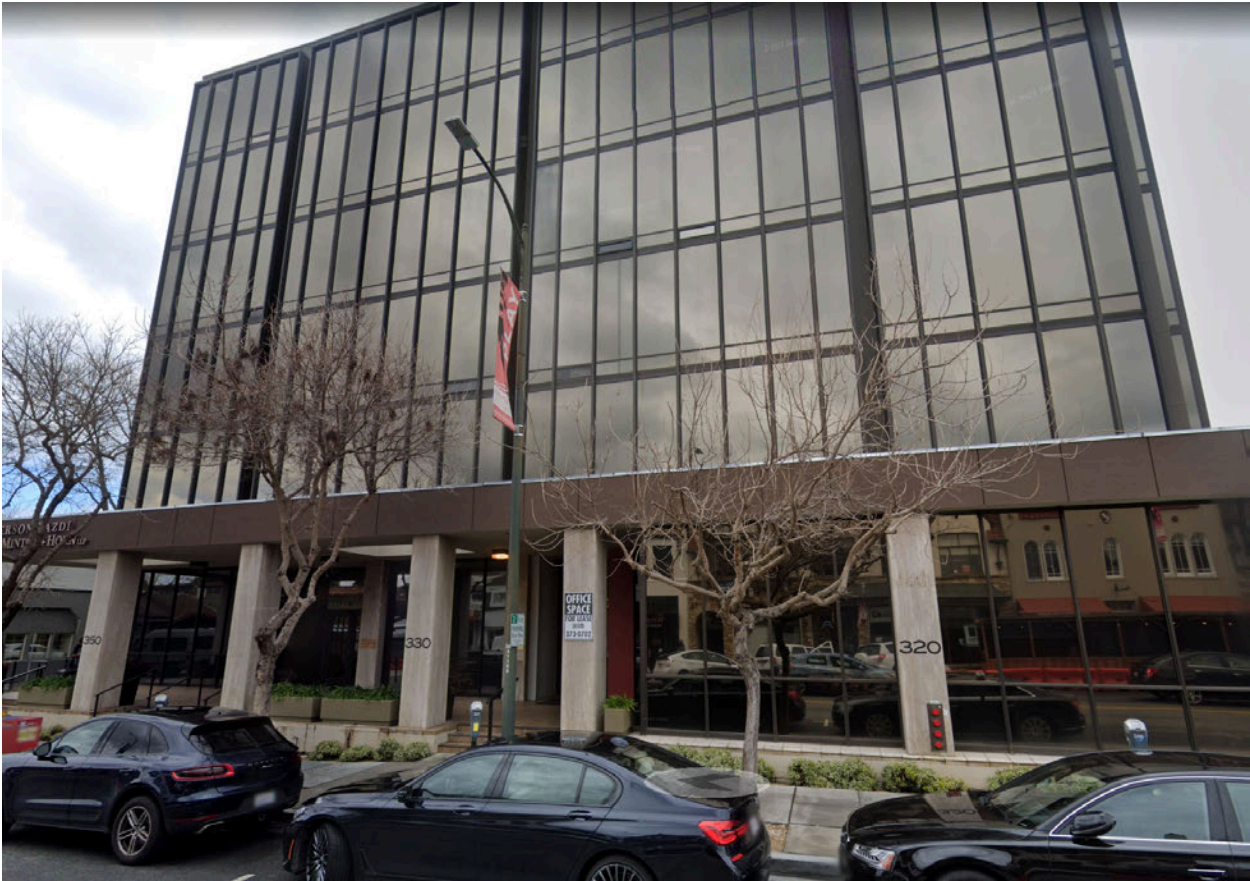
FAIL. Burlingame. Side Street. Taller buildings allowed without pedestrian focus.
