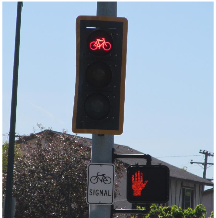
A traffic signal specific to bicycling. Dedicated bike signals, like this one at Story Road and Hopkins Drive, are a useful tool for biking through protected intersections. Credit: City of San José
