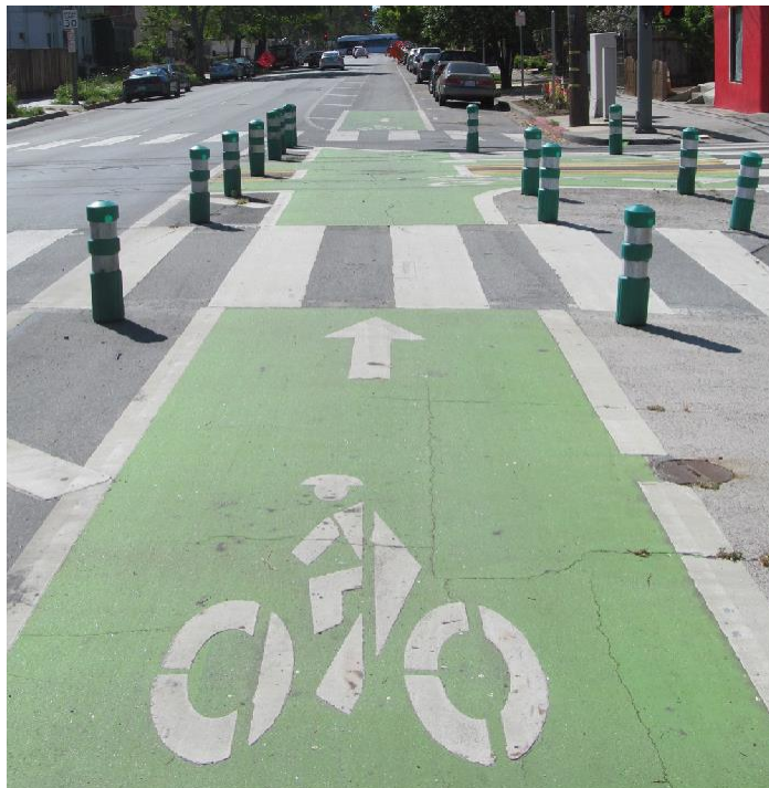
A painted bike lane with green bollards. Great intersections, such as this one at 10th and St John Street, make up the future of bikeways. Credit: City of San José
