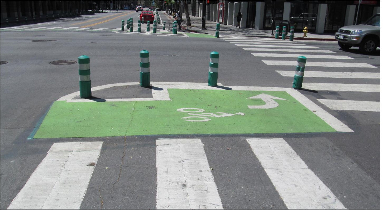
A green-painted box protected by bollards. Two-stage left-turn bike boxes, such as this one at 4th and San Carlos Street, is helpful for navigating through intersections. Credit: City of San José
