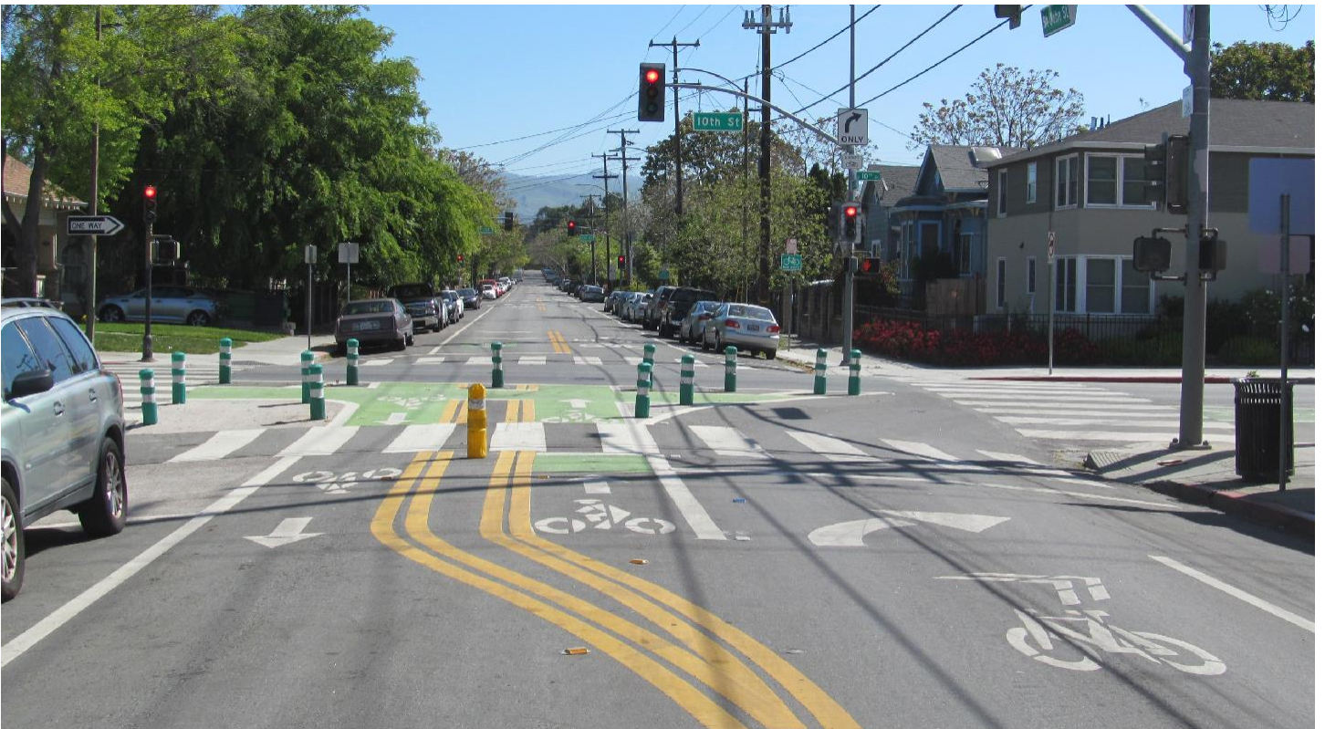
An intersection with green paint and bollards that diverts cars one way and allows bicyclist to ride through. Bike boulevard diverters, like at 10th and St John Street, maintain low volumes of cars on low-stress bike boulevards. Credit: City of San José
