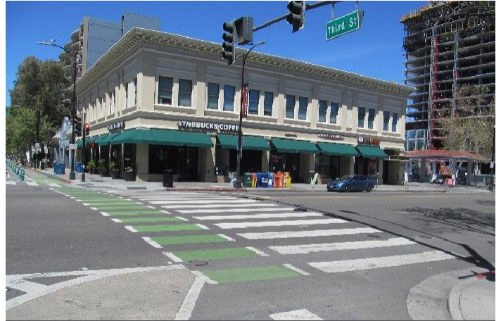
Green painted bike lane markings through an intersection, like those at 3rd and E Santa Clara Street, are part of bikeway designs at intersections. Credit: City of San José
