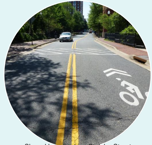
Shared lane marking St John Street
