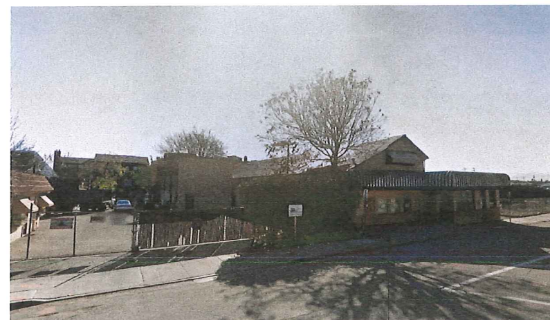
Project Location View B
