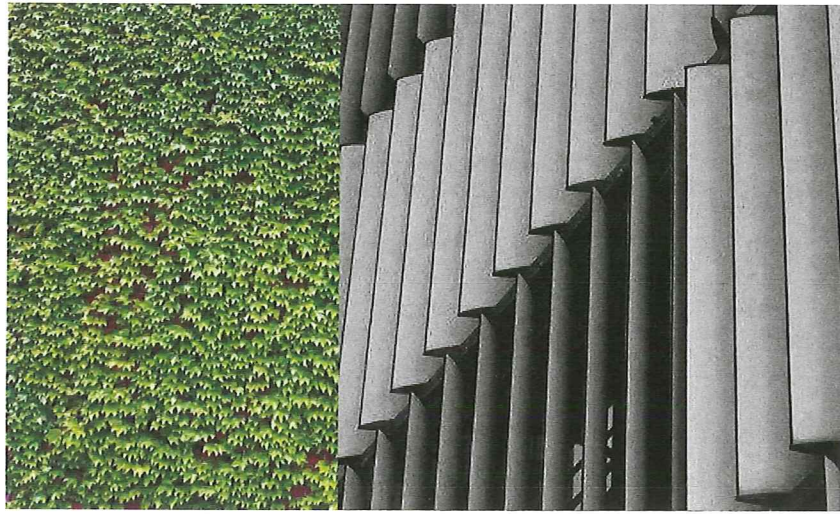
PARKING STRUCTURE GREEN WALL AND METAL GRILLE
