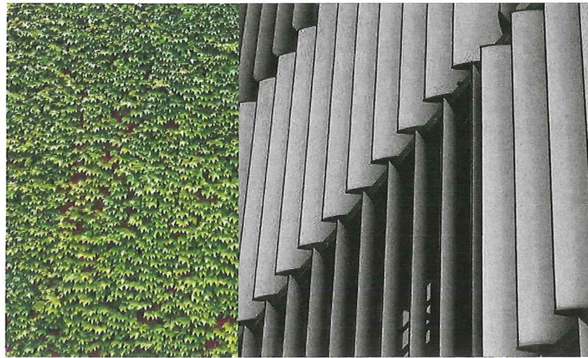
PARKING STRUCTURE GREEN WALL AND METAL GRILLE
