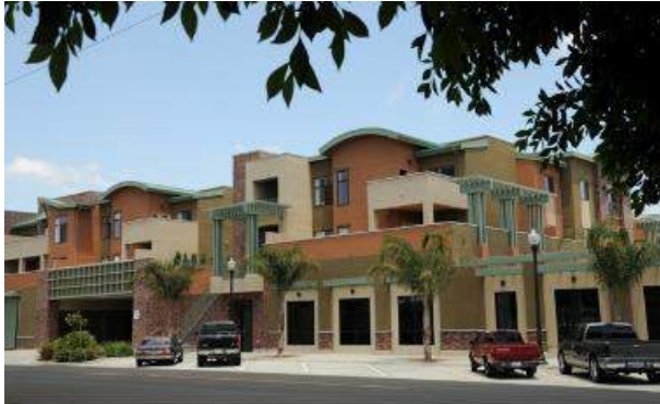
Colonial House Apartments, Oxnard
