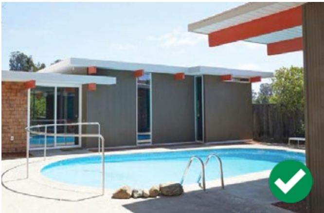
Figure 56: An ADU with a roof form and detailing inspired by the original Eichler house on the lot. Source: Eichler Network.
