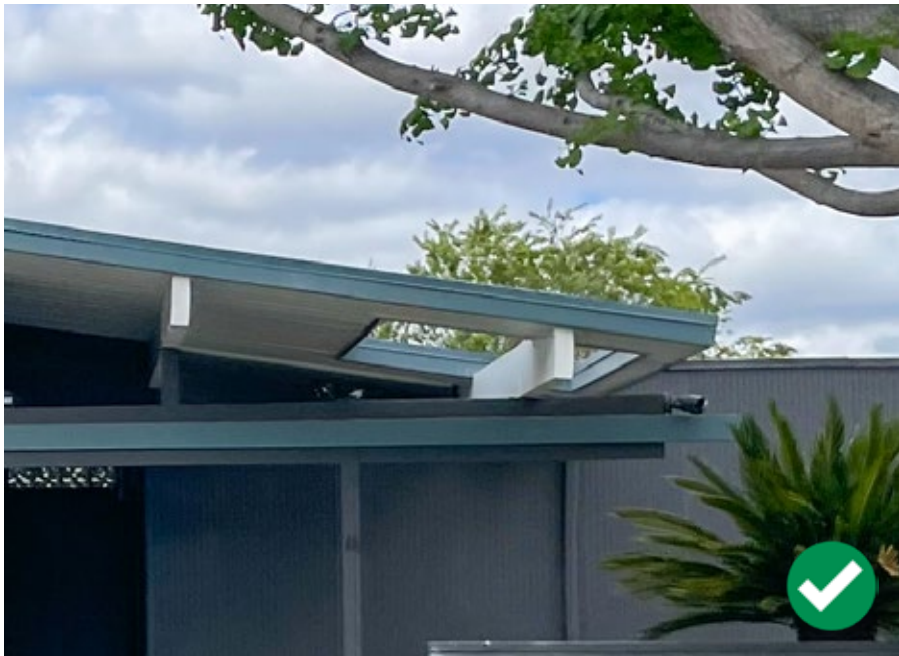
Figure 10: Preserve roof openings.
