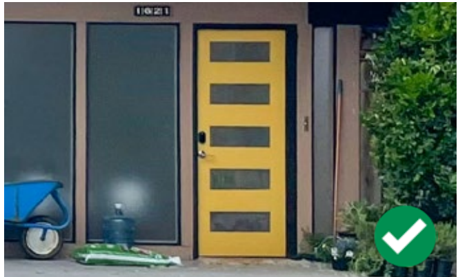
Figure 31: An appropriate replacement front entry door with a flat planar surface and rectilinear glazing.
