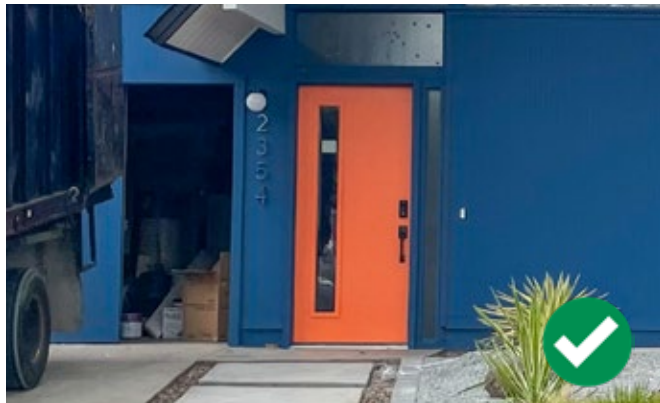
Figure 29: An appropriate replacement front entry door with a flat planar surface and rectilinear glazing.
