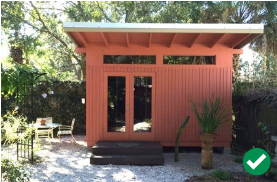
Figure 58: An ADU with a shed roof and vertical wood siding, which are compatible materials with Eichler homes. Source: Historic Shed.
