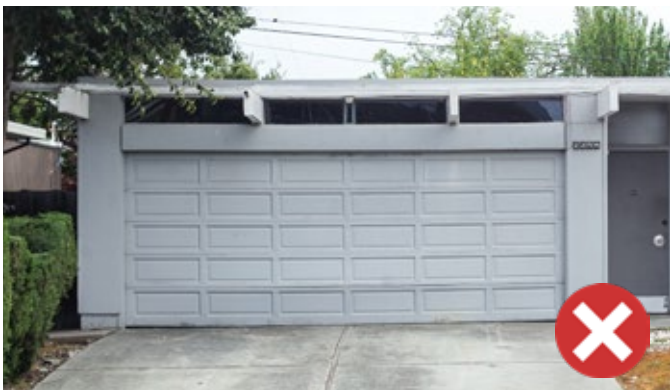
Figure 24: Paneled garage doors are prohibited.
