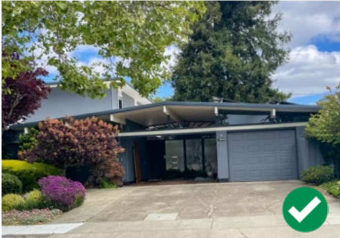
Figure 44: This addition is set back from the front facade with a floor height that is lower than the original house.
