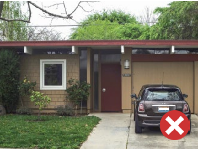
Figure 37: Adding new windows at front facades is prohibited.
