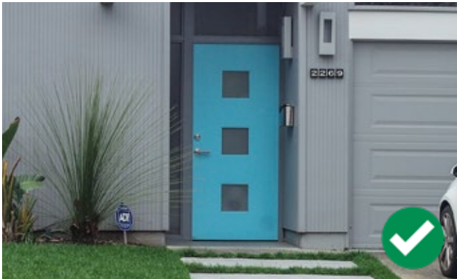
Figure 30: An appropriate replacement front entry door with a flat planar surface and rectilinear glazing.
