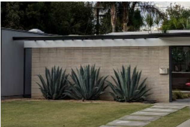
Figure 17: Original rectangular concrete block cladding.
