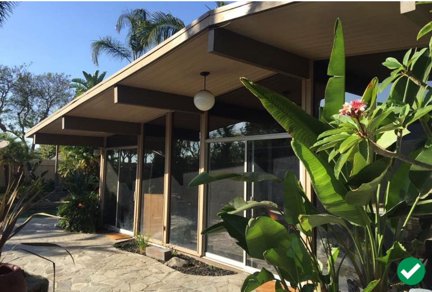
Figure 40: Original full-height fixed windows and window walls at secondary and rear facades shall not be infilled. Photo courtesy of Sally Zarnowitz.
