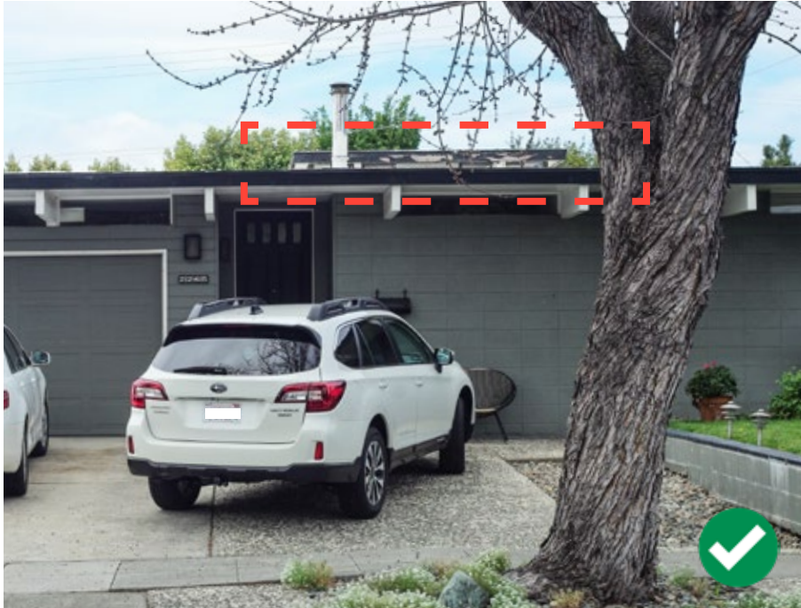
Figure 48: This atrium cover is low and has a flat roof like the original house.
