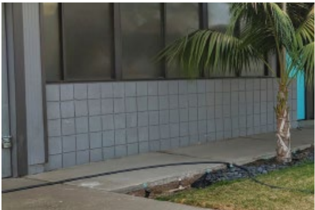
Figure 16: Original square concrete block cladding.
