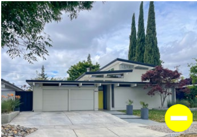
Figure 45: This addition has a skillion roof form, cladding, and windows that are allowed. However, the design would be improved by setting it further back from the front facade and reducing the floor heights.
