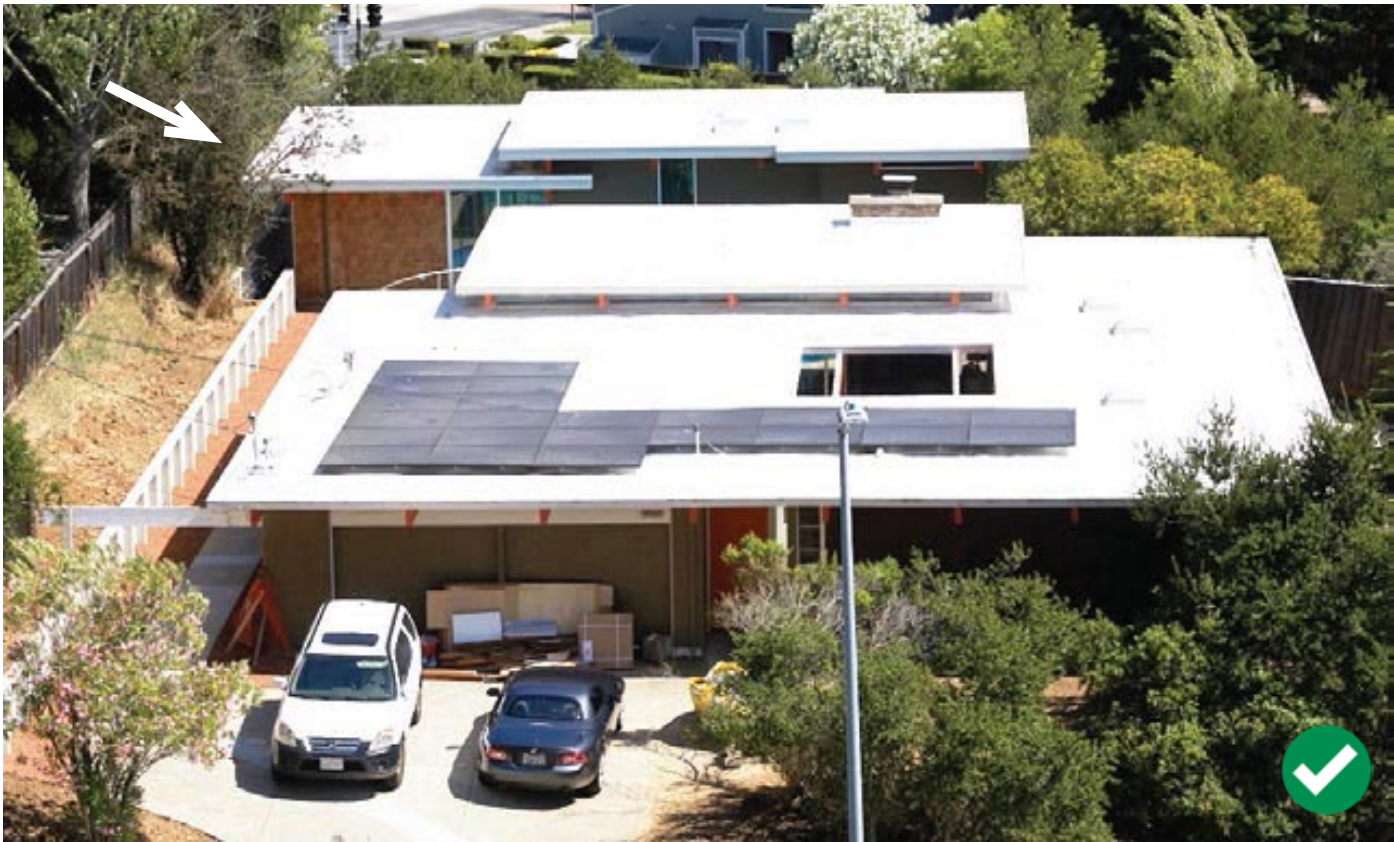
Figure 55: A rear ADU (indicated by white arrow) that has a similar height and roofline to the Eichler house at the front of the property. Source: Eichler Network.
