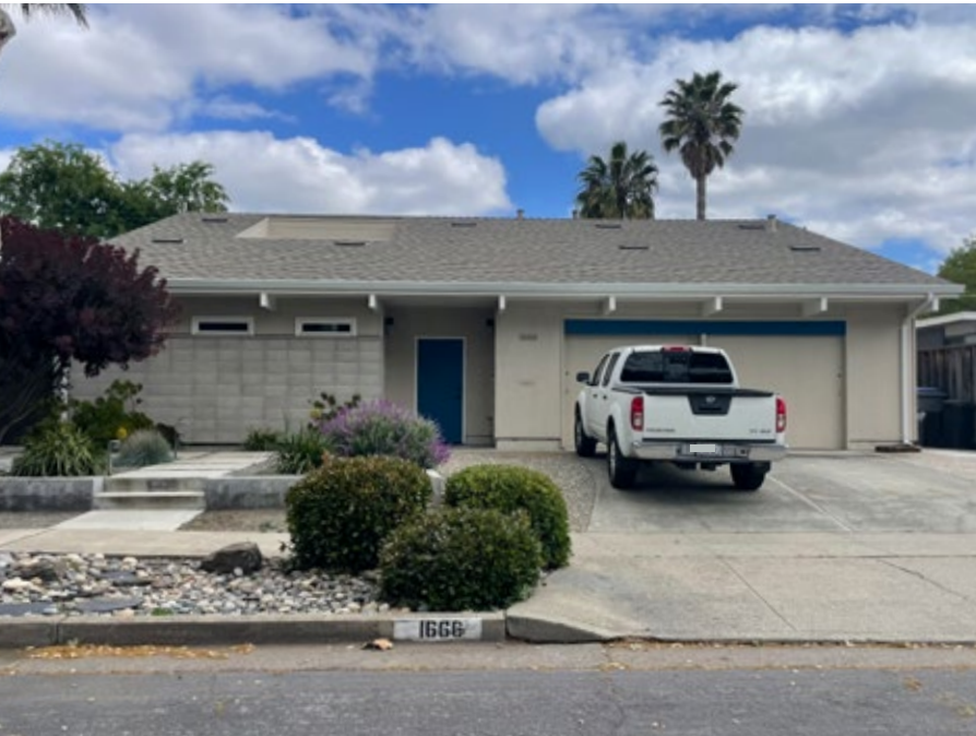
Figure 50: These altered Eichler residences have non-original roof forms and would be considered non-contributing properties.
