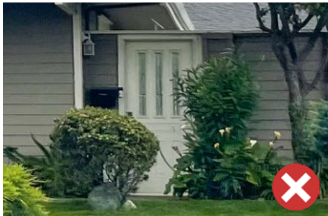
Figure 33: Replacement front entry doors with beveled art glass are prohibited when visible from the street.
