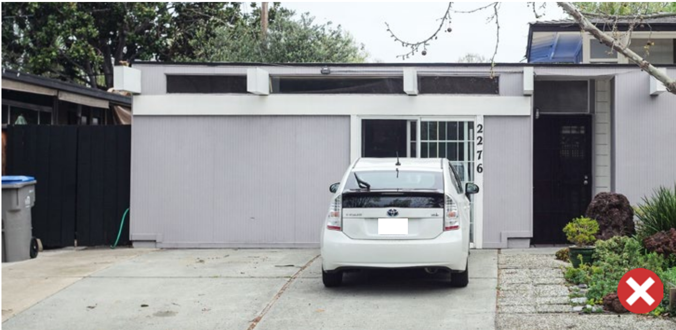
Figure 27: Adding new door openings at the front facade is prohibited.
