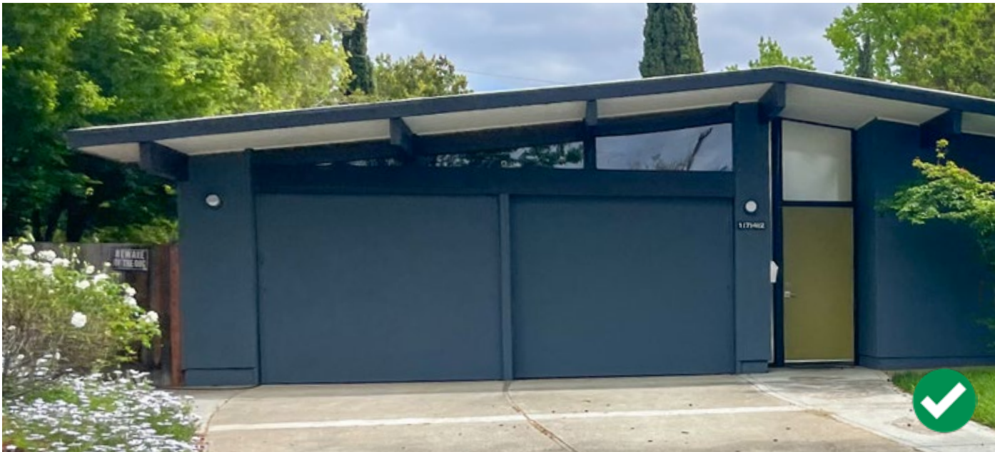
Figure 21: Preserve and maintain original garage doors.
