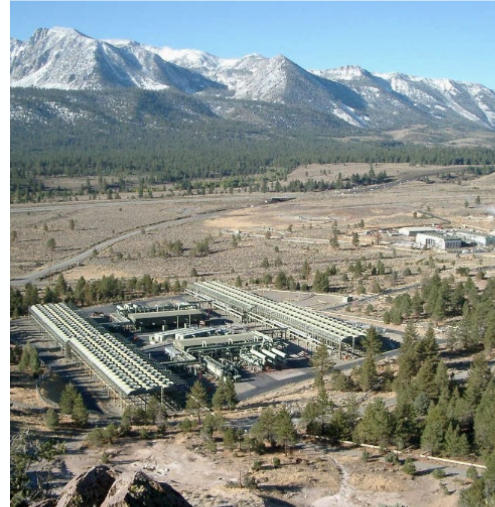
Ormat's Mammoth geothermal facility in CA
