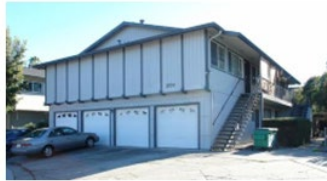
Low-Rise Multifamily Building
