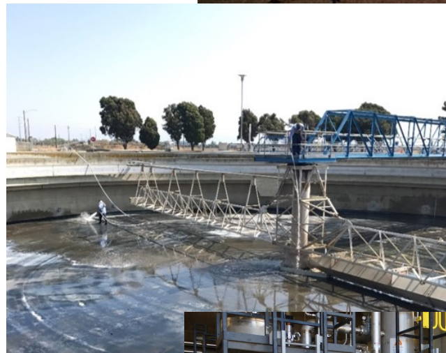
Facility-Wide Water System Improvements
