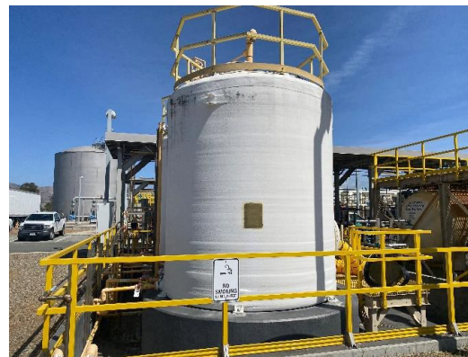
Tank Rehabilitation and Inspections
