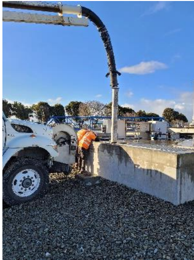
Hydroflushing and inspection of plant influent pipe
