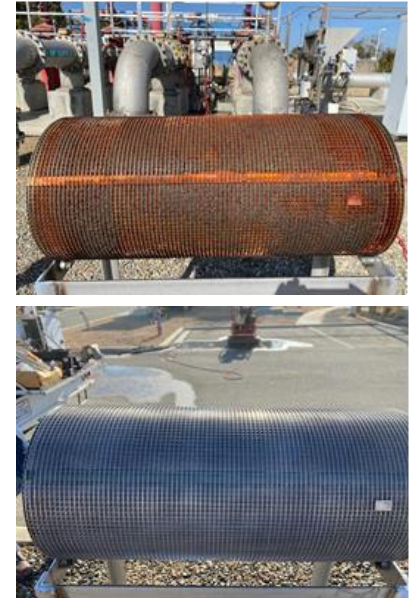
Autostrainers rehabilitation and cleaning
