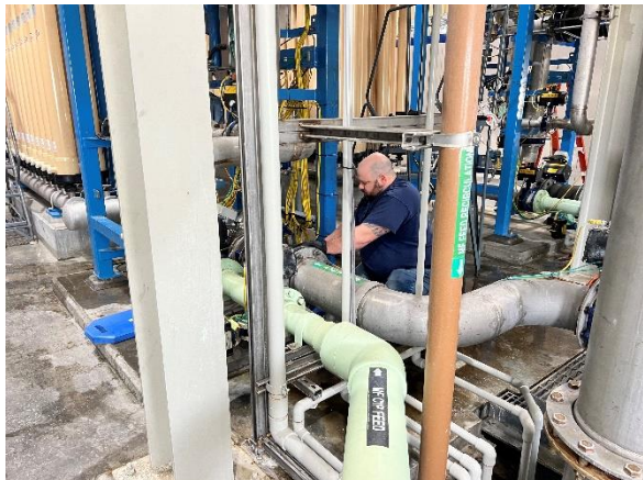
MF rack valve replacement
