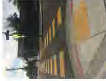
6 ADA CURB RAMP AND CROSSWALK SCALE: NTS
