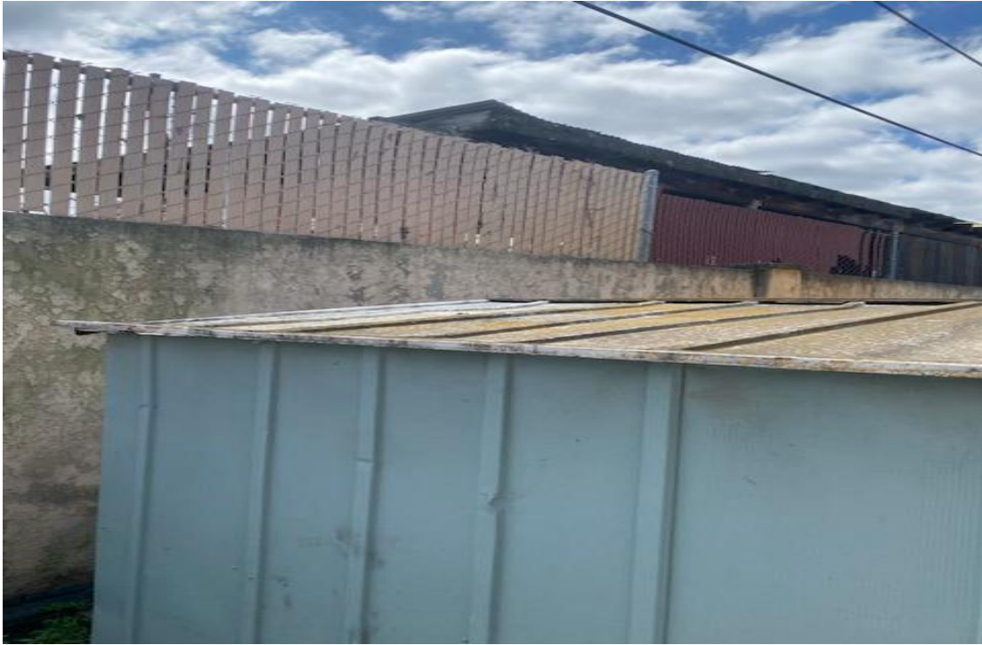
Soundwall that separates the Walnut MHP from the South Yard
