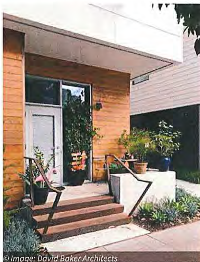
Fig. 3.15 Occupied front porch at least four feet deep and six feet wide to make room for outdoor furniture and seating.
