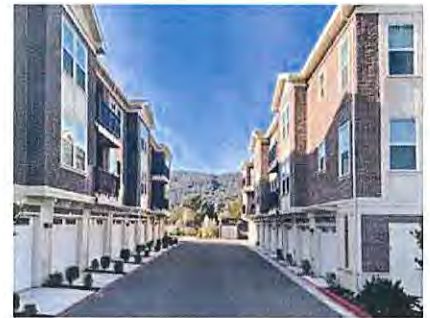
Fig. 2.8 Locate garages, parking pads, and driveways for individual residences on secondary streets , alleys, or private streets .
