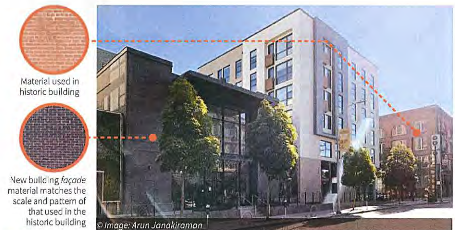
Fig. 3.9 Materials for street-facing façade of new developments similar to the adjacent historic building.
