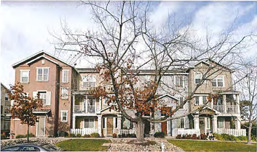
Fig. 5.4 A four-plex with all unit entrances facing the street. Some units have front yard patios whereas others have a recessed unit entrance or a front door with a projecting awning for weather protection.
