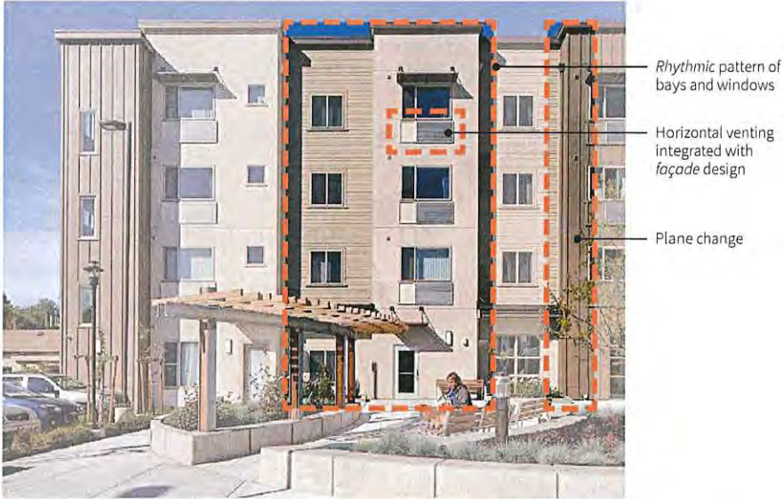
Fig. 3.22 Articulate façades and create a rhythm of architectural features such as bays and windows.
