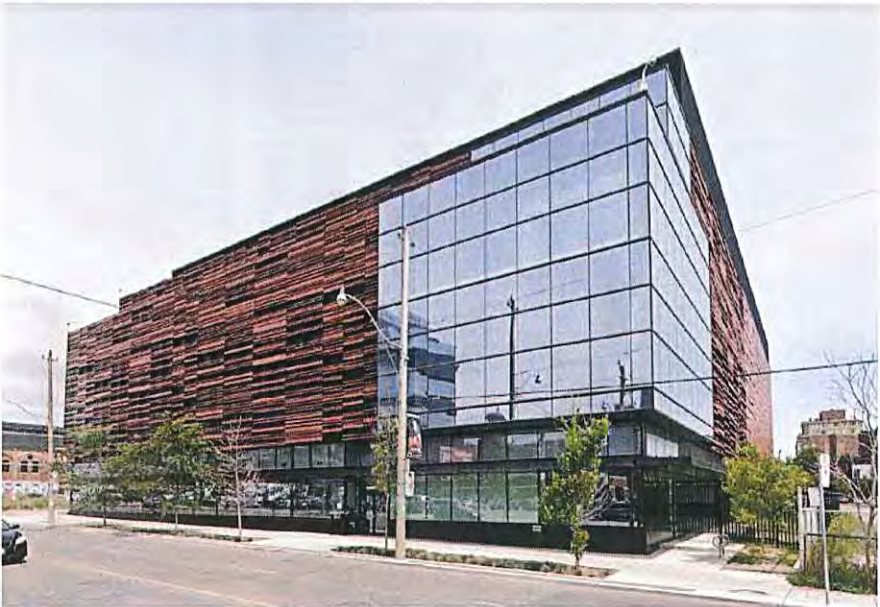
Fig. 5.43 A data center in an urban area with façade articulation , special corner treatment and upper floors setback from the street.
