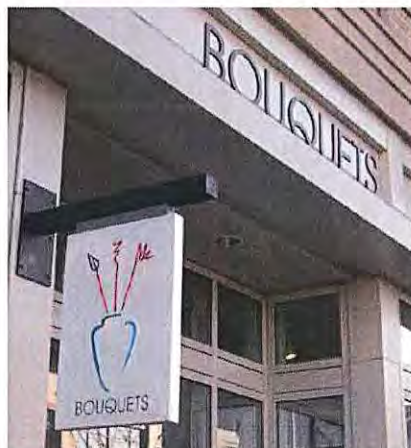
Fig. 3.55 Blade or fin signage reflects the character and image of the use.
