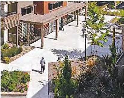
Fig. 2.40 LID planters help manage site stormwater runoff as well as run-off from building roofs using downspouts.
