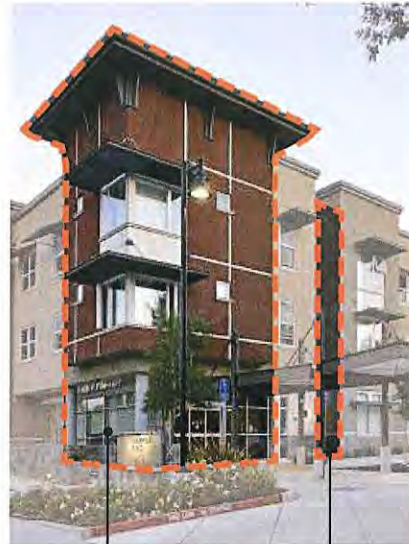
Articulated corner with exaggerated roof element
