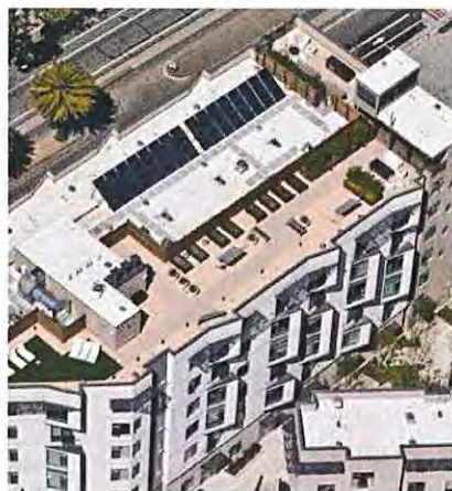
Fig. 3.31 A flat roof can be used for a combination of renewable energy systems such as photovoltaic solar panels and low-maintenance landscaping.
