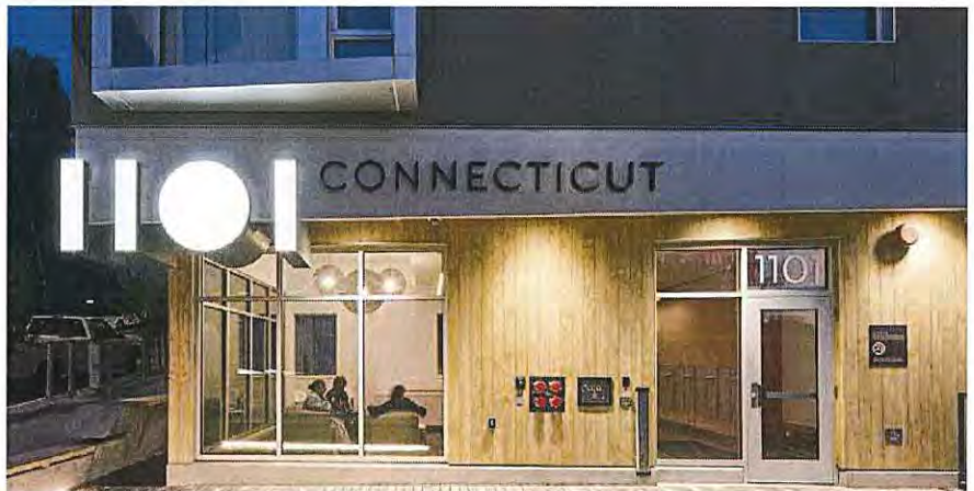
Fig. 3.54 Illuminated awning sign placed at entry canopy to identify the building address and emphasize building corner.
