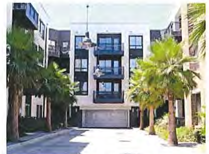
Fig. 2.9 Locate driveways on secondary or less prominent streets away from public open spaces and street intersections.
