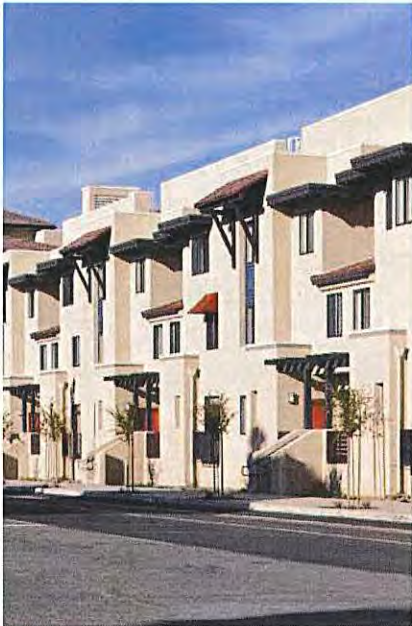
Fig. 4.9 Frequent residential entrances along the street to create eyes-on-the-street.
