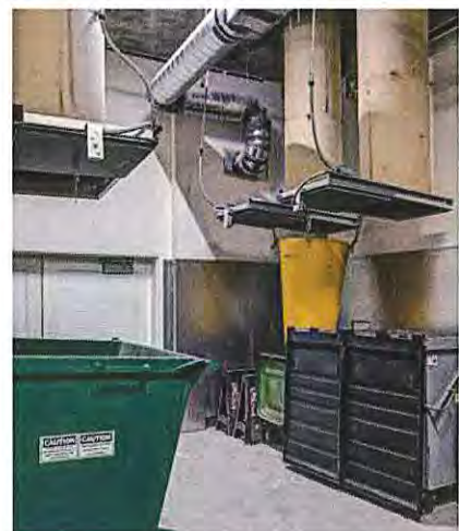
Fig. 2.12 An on-site solid waste area located inside a building.
