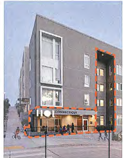
Articulated building corner with public plaza
