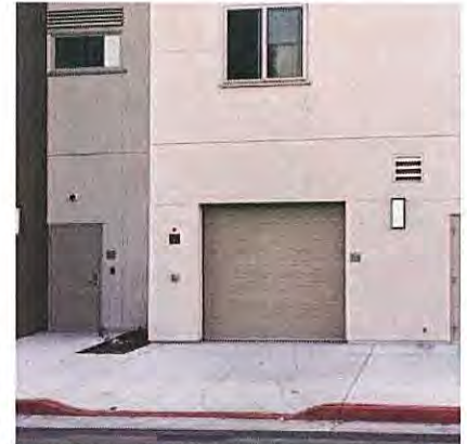
Fig. 3.20 Locate and design access to utility areas and solid waste rooms away from building entrances and towards the rear or side of buildings.
