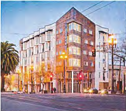
Fig. 5.16 Mid-rise mixed-use building with façade articulation, window patterns, varying roof heights, and special corner treatment.
