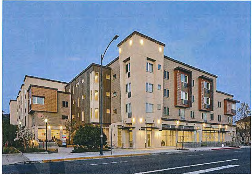
Fig. 3.51 Ornamental and architectural lighting at the ground floor highlights the features of buildings and creates uniform lighting conditions along the perimeter.
