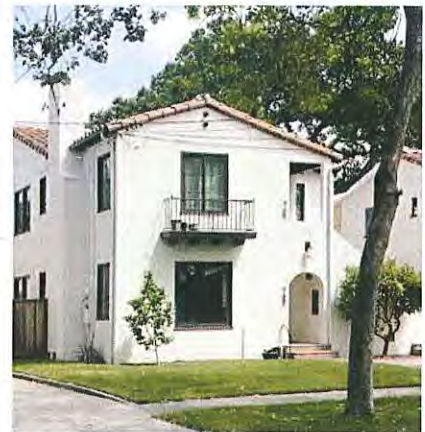
Fig. 5.3 Example of duplex configuration where one unit is located on the ground floor with direct access from the street and the other is located on the second floor with a walkway from the street to the staircase.
