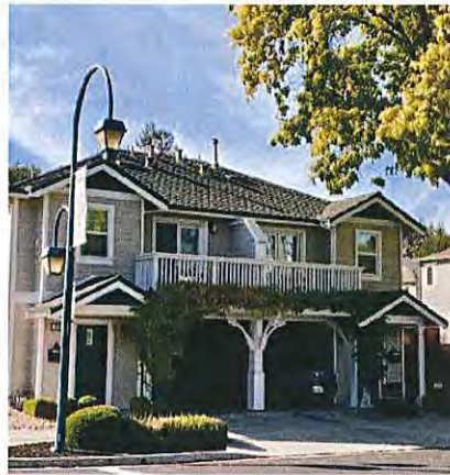
Fig. 5.2 Single-family house converted to duplex by adding an additional floor, splitting the building into two units with entrances for each unit located on the ground floor on each side of the building frontage .
