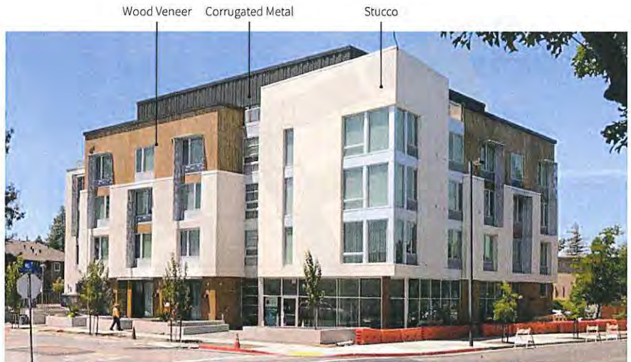
Fig. 3.48 Use contemporary or traditional materials to define a base, middle, and top for buildings and to highlight corner elements.
