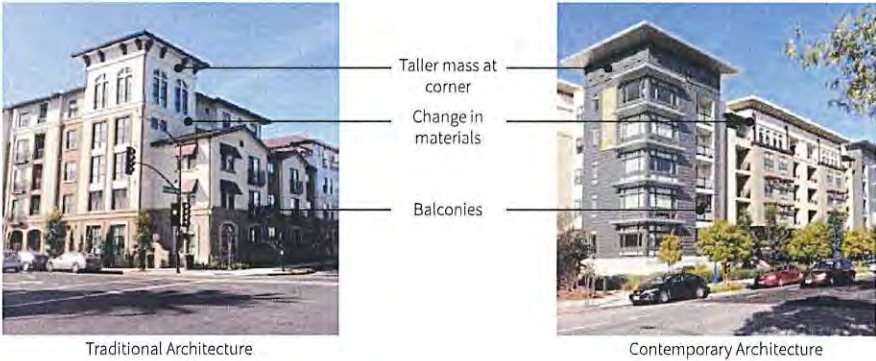
Fig. 3.23 Similar design elements such as bays, balconies, and window treatments can be used with different architectural styles.
