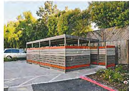
Fig. 2.10 Screen on-site solid waste and utility areas located outside the building.
