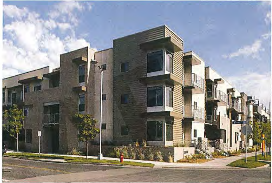
Fig. 5.12 Façade articulation, special corner treatment, decks and balconies, recessed parking garages, and residential entrance stoops accessible from the street create smaller masses and bring this low-rise multifamily residential building to a human scale .
