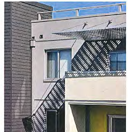
Fig. 3.39 Vertical and horizontal sunshades and awnings create interesting shadow patterns and reduce solar heat gain.
