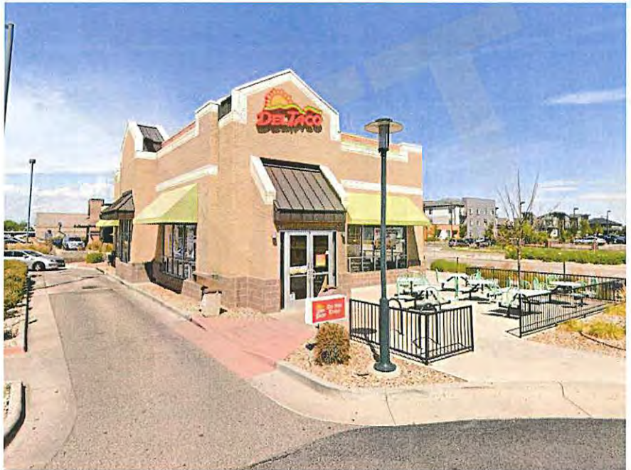
Fig. 5.59 A drive-through outside General Plan Growth Areas and a part of a commercial corridor. The building is placed towards the street and designed with an architectural idea similar to the adjacent buildings. The drive-through provides enough space behind the building for several cars to line up at the pick-up window.
