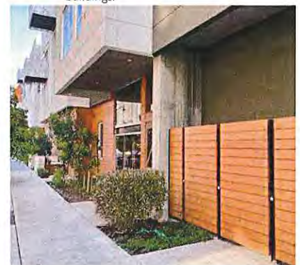
Fig. 3.21 Provide covered solid waste and utility enclosures when outside of buildings and screen them from the public realm .
