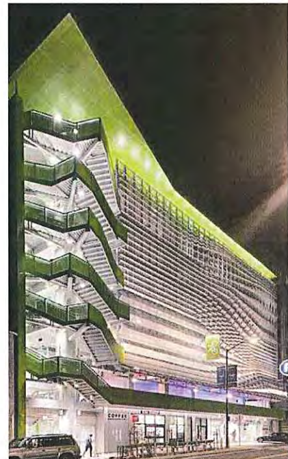
Fig. 3.42 Conceal all ramped floors from street view and line the ground floor façade with active uses .
