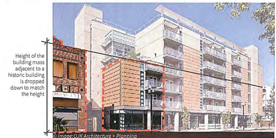
Fig. 3.10 Building massing stepped down adjacent to a historic building to transition from the scale of the development to the scale of the historic building.
