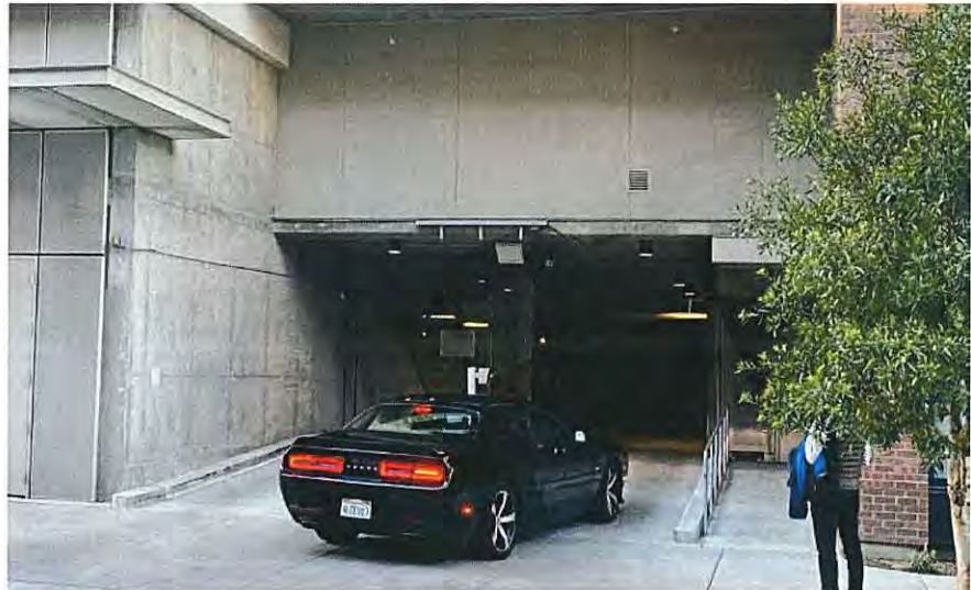
Fig. 3.17 Driveways recessed into the building façade protect pedestrians on sidewalks from incoming and outgoing vehicular traffic.
