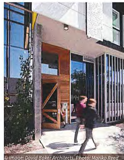
Fig. 3.16 Building entrance along the public realm recessed to provide weather protection and avoid bumping into pedestrians walking by.
