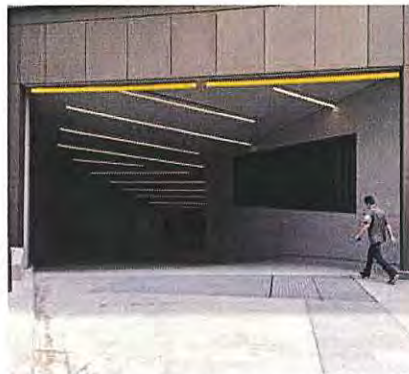
Fig. 3.41 Provide flare-out openings at garage entrances for enhanced driver visibility and pedestrian safety.
