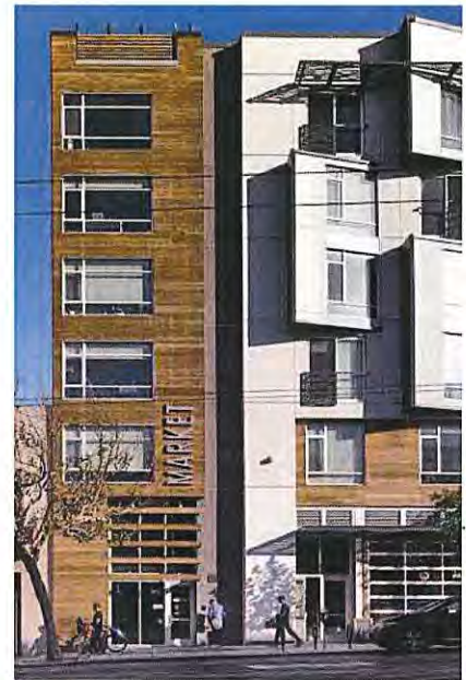
Fig. 2.6 A convenient and clearly-visible pedestrian and bicycle entrance.
