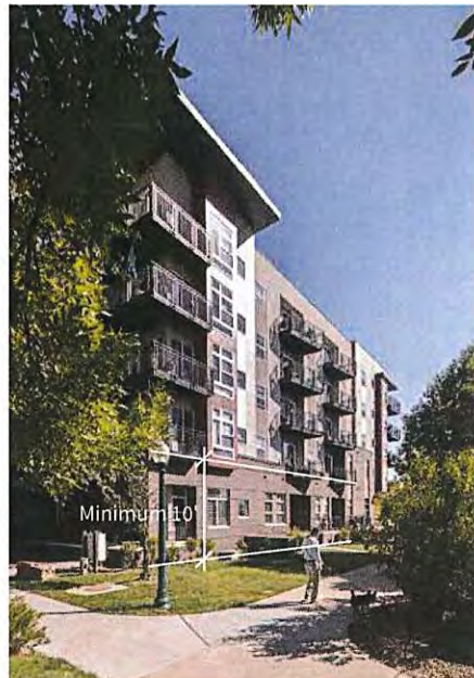
Fig. 2.23 Articulate building façades along paseos and provide a minimum of 10 feet height clearance between paseos and building elements like balconies, trellises, and sunshades .
