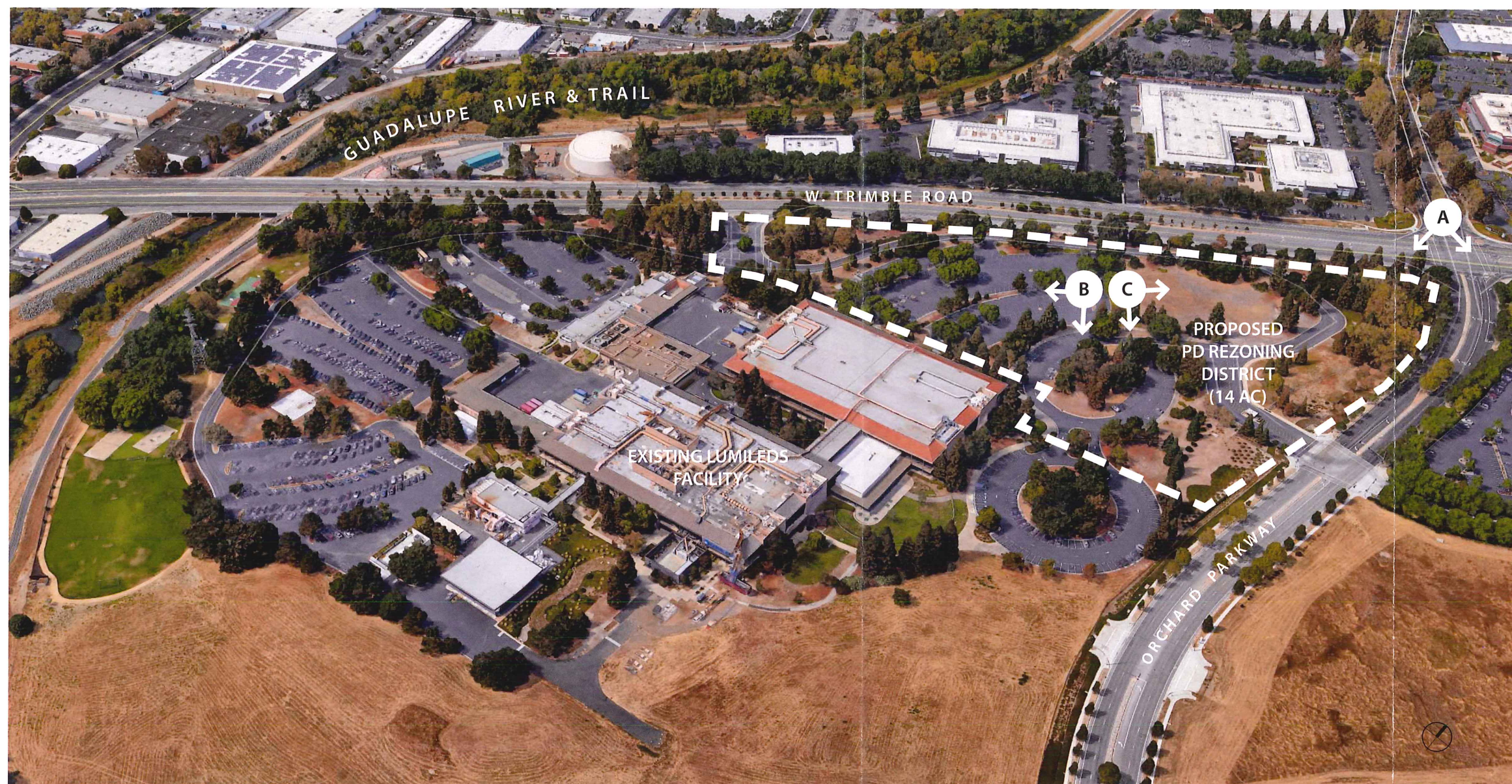
AERIAL VIEW LOOKING NORTHWEST
