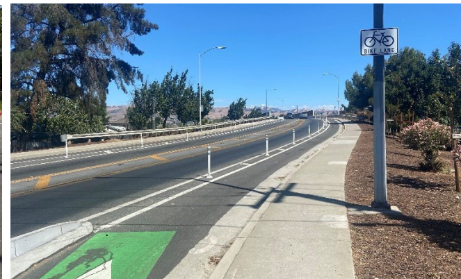
Figure 7: Protected bikeway over Highway 101.
