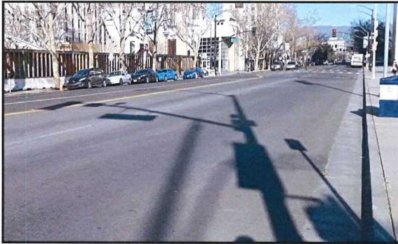
Good (PCI 100 to 70) – Santa Clara St. PCI 91
