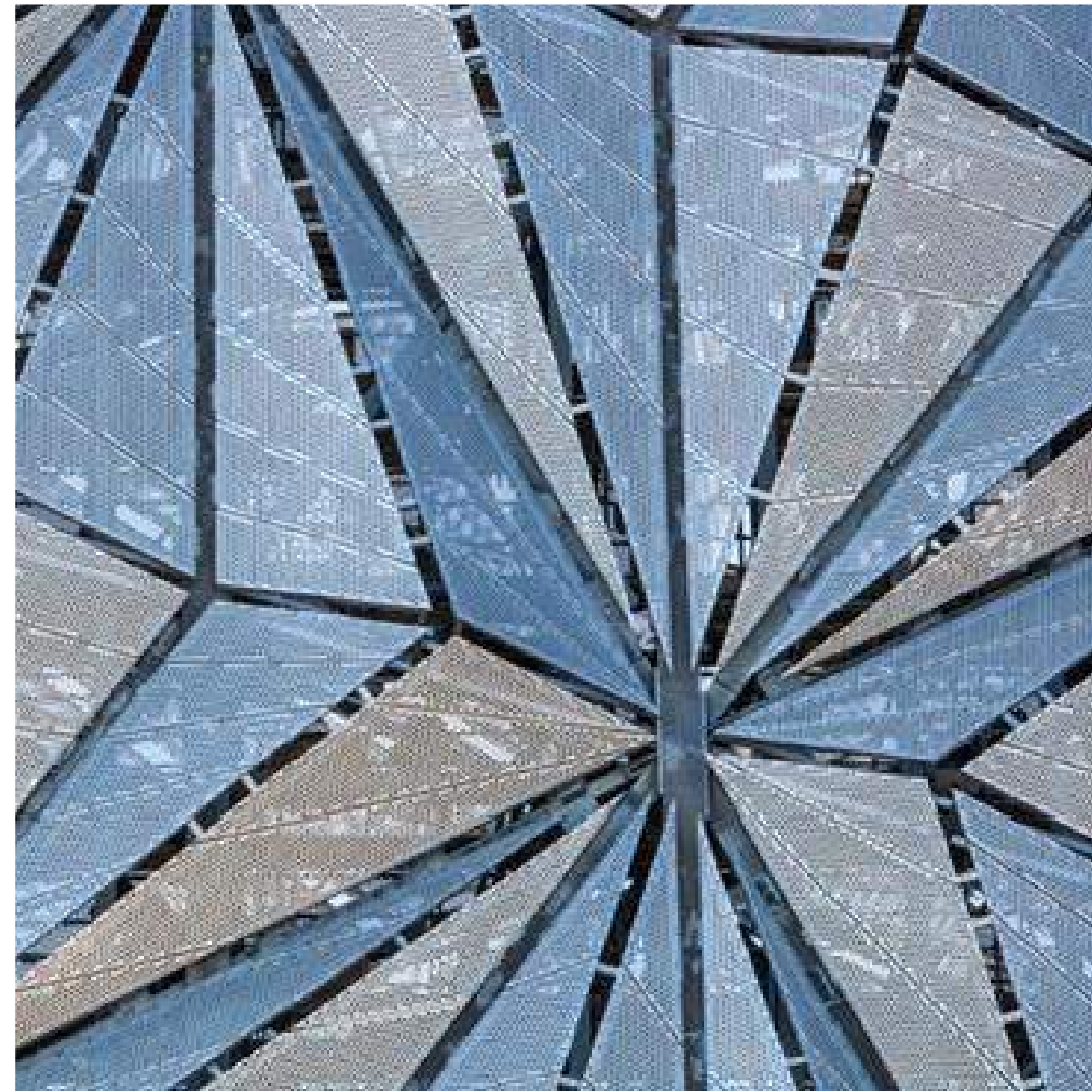
(B) PERFORATED METAL Canopy panels - Daytime photograph of Greenwich Energy Centre / C.F. Moller Architects, expresses some translucency as well as warm and cool tones.
