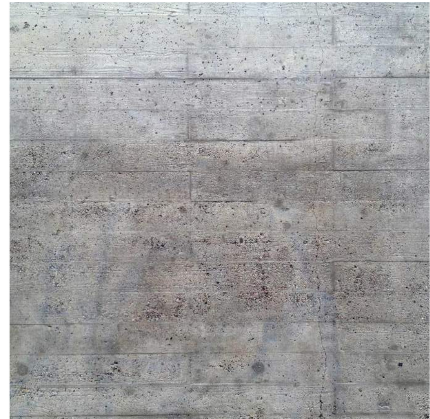
BOARD FORMED CONCRETE Walls facing the pavilion and stage (South elevation)
