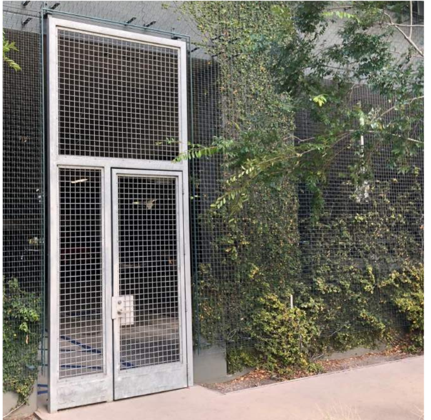
FENCING AND GATES Exterior gates to include similar screening without plant growth.
