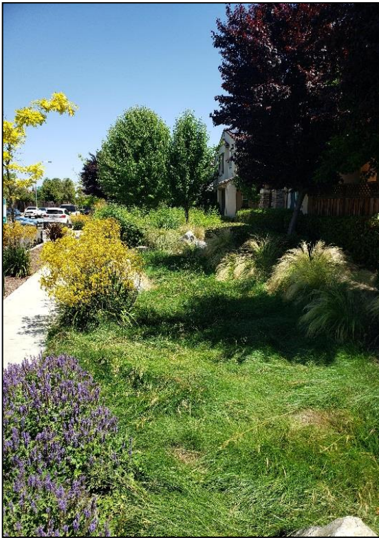
Bioretention installation in a residential area.
