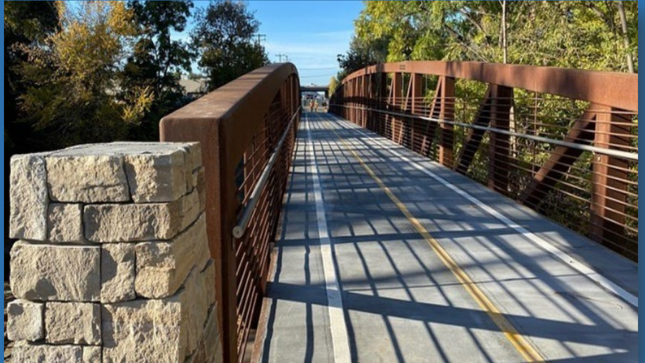
Los Gatos Creek Trail/Three Creeks will soon connect over the new Three Creeks Trail Bridge.
