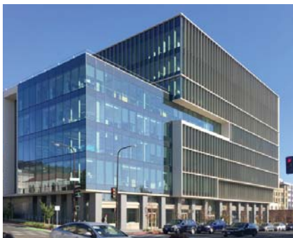
DO - Vary fenestration by building facade , placing windows to take advantage of solar conditions and views to the nearby ground level Public Realm .
