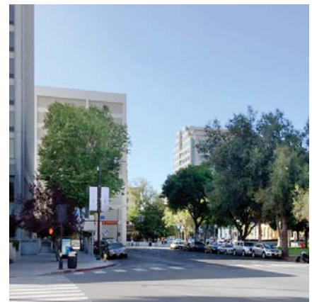
DO NOT - A tower southwest of a plaza may create large areas of shade, reducing the ability of users to choose the amount of shade based on comfort.
