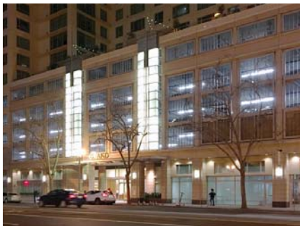
DO and DO NOT - This parking garage allows harsh light to intrude onto the street. However, the building also uses creative Podium Level lighting to create distinction (see Section 4.4.9.a).
