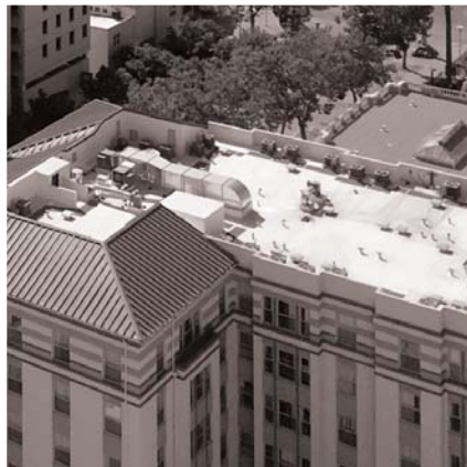
DO NOT - A cluttered, disorganized-appearing rooftop diminishes views from nearby buildings.
