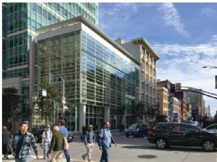
DO - A lower massing element creates a transition to shorter buildings nearby.
