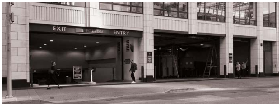
DO NOT - Adjacent entry and loading doors create a long zone where pedestrians are in danger from vehicles and with no Active Frontage .
