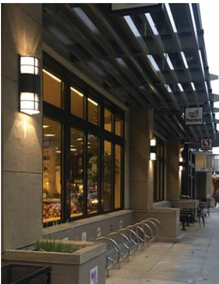
DO - Provide frequent light fixtures to create additional, more pedestrian-scale lighting than that from street lamps.
