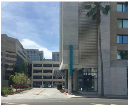
DO - Place a parking garage behind the main building to reduce its effect on the Streetscape .
