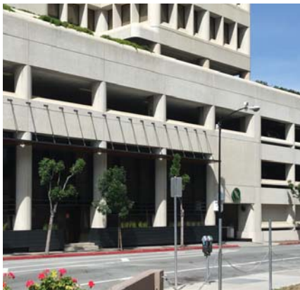
DO - Place vehicular entries away from intersections and on lower status streets to avoid disruption of primary frontage .
