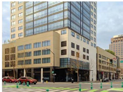
DO - Treat the facade of an exposed parking garage with materials and design similar to the rest of the building and extend the tower facade to ground level (see Section 4.3.1).
