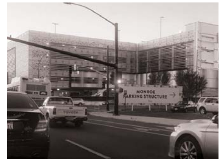
DO NOT - Exposed parking diminishes the Public Realm even if the garage is decorated.
