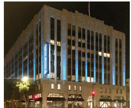
DO - Use Wall Washing to accentuate the Podium Level . If lights are pointed upward, avoid spilling extra light away from the building.
