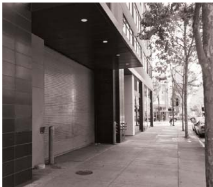
DO NOT - A service entry can create poor conditions on the sidewalk.
