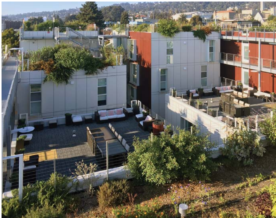
DO - Green roofs (including food production) and Roof Decks for residents' use top the 3rd, 4th, and 5th floors of Garden Village in Berkeley.
