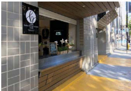
DO - Small retail spaces such as these on the San Pedro Market Parking Garage create Active Frontage and reduce the length of a Blank Wall .
