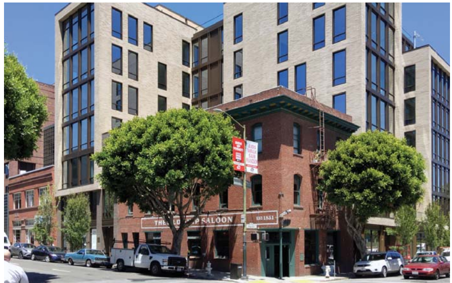
DO - The new building at rear responds to Historic Adjacency through materials and fenestration.
