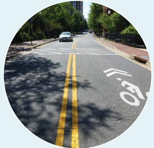
Shared lane marking St John Street
