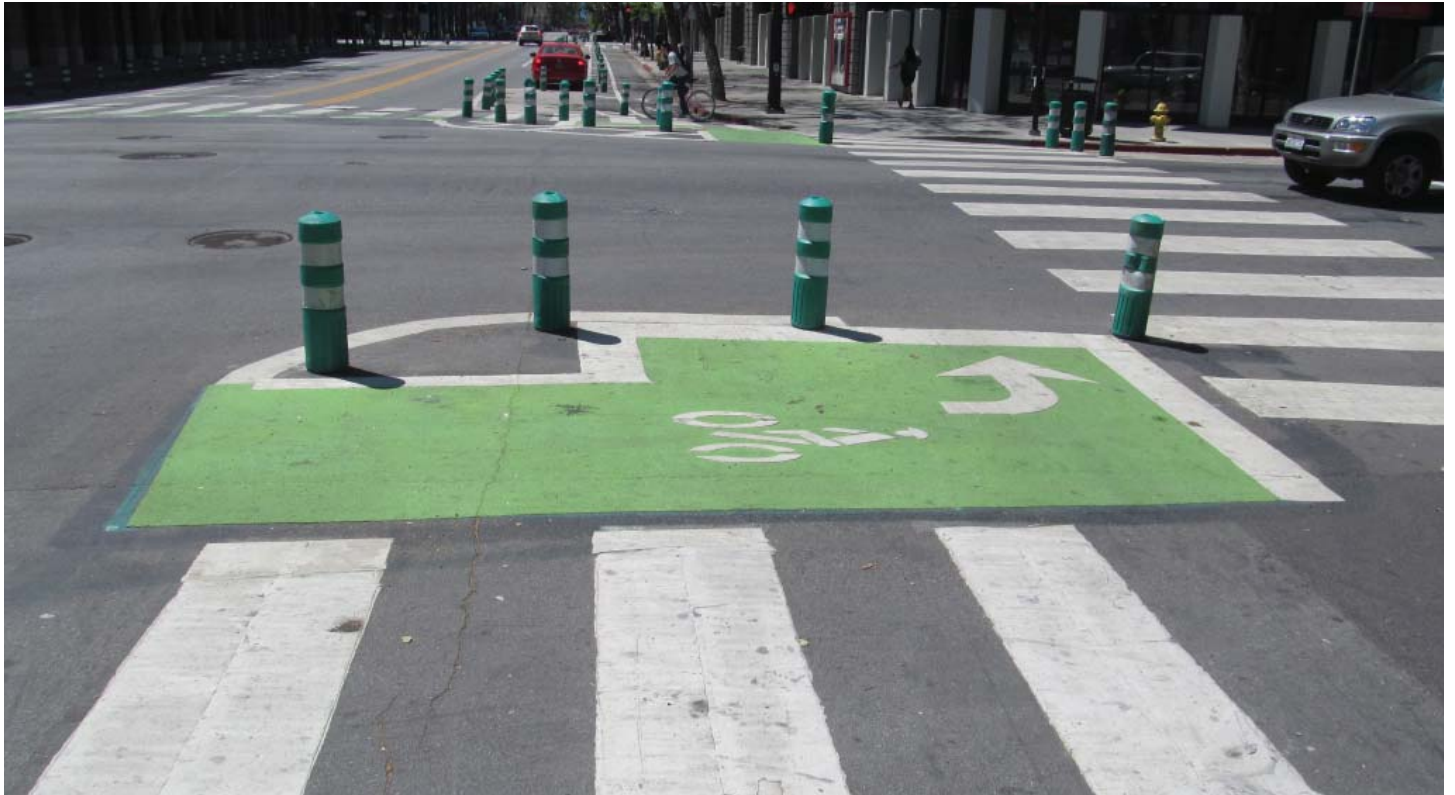
A green-painted box protected by bollards. Two-stage left-turn bike boxes, such as this one on San Fernando at 4th Street, is helpful for navigating through intersections. Credit: City of San José
