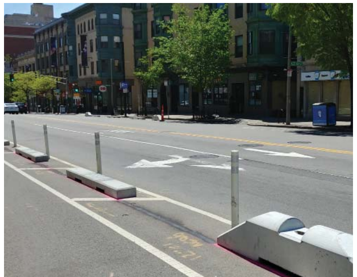
Pre-cast concrete curbs provide a higher quality buffer between the bikeway and vehicle traffic at a slightly higher cost.
