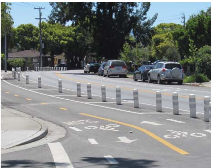
Flexible plastic posts provide physical separation between the bikeway and vehicle traffic at a relatively low cost.
