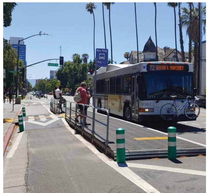
To minimize conflicts between transit riders, bike riders, and bus operators, VTA and the City of San José collaborate to build bus boarding islands, as shown in this photo.
