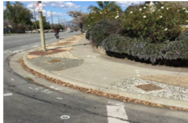
Missing – No ramp present
