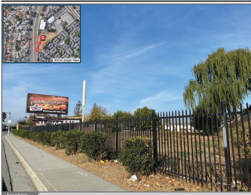
Figure 1 – The existing monopole and radome.
