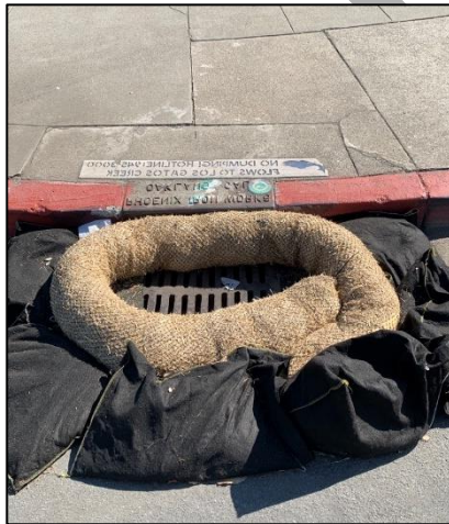
Effective BMPs installed at construction site.
