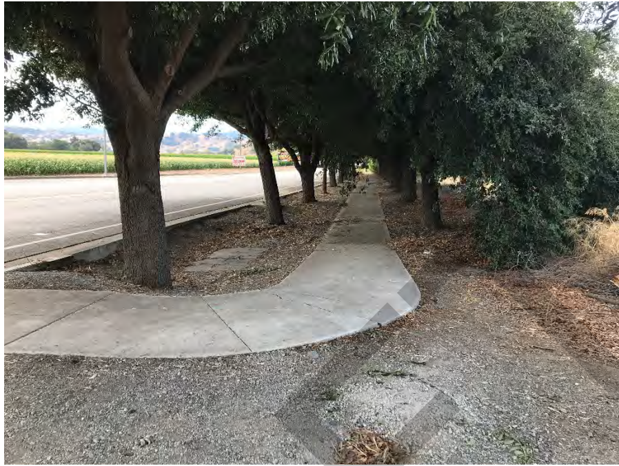
Eastern terminus of sidewalk along the north side of Bailey Avenue.
