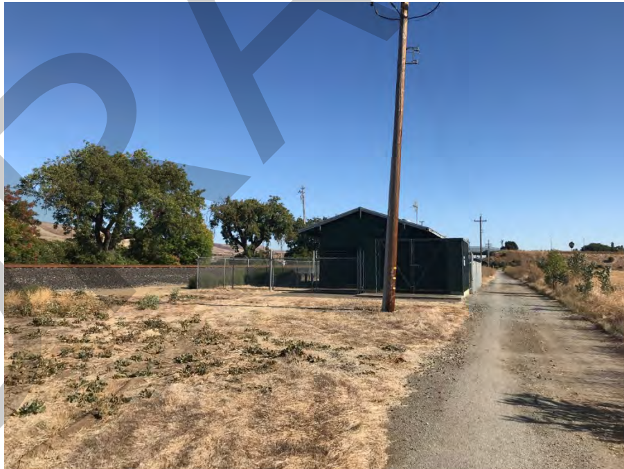
North side of municipal pump house #22-1B and Southeast Perimeter Road
