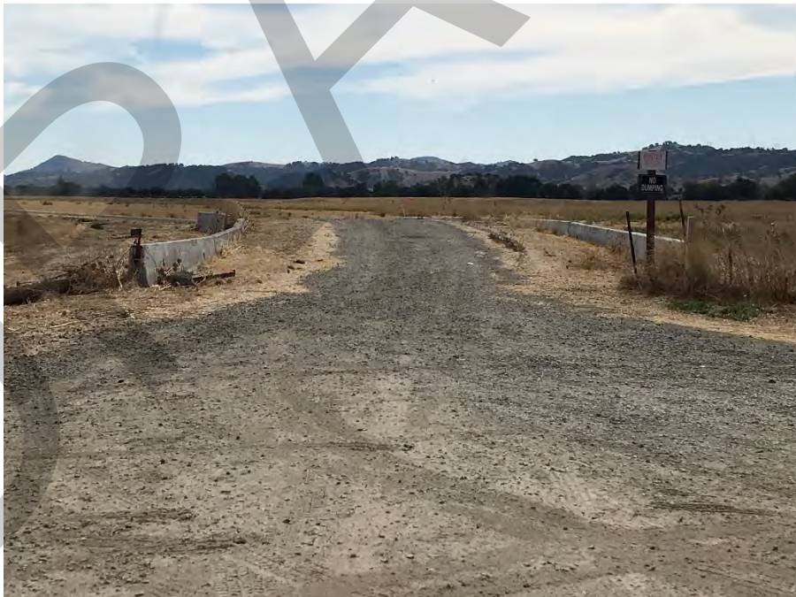
Entrance to Calpine Road off Blanchard Road.
