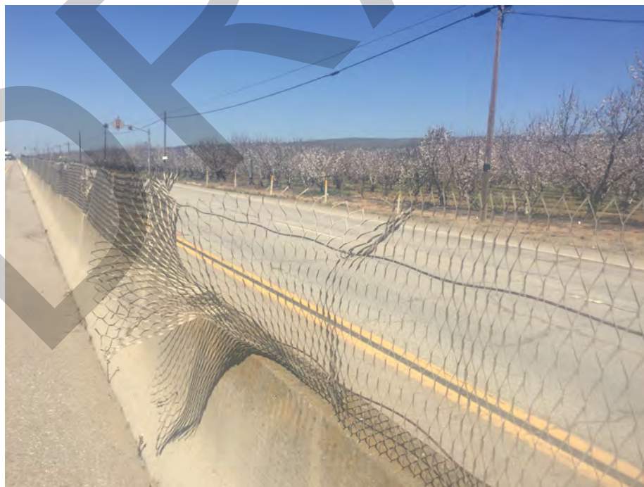
Median barrier on Monterey Road. Photo by Stephi Matsushima.
