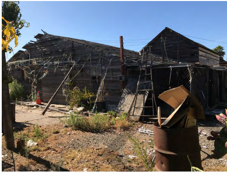
Southern portion of the Emado Compound. South side of the barn.
