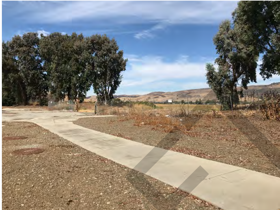
Chain link gate and fencing and steel barrier gate (opened) at southern turnout along Santa Teresa Boulevard.
