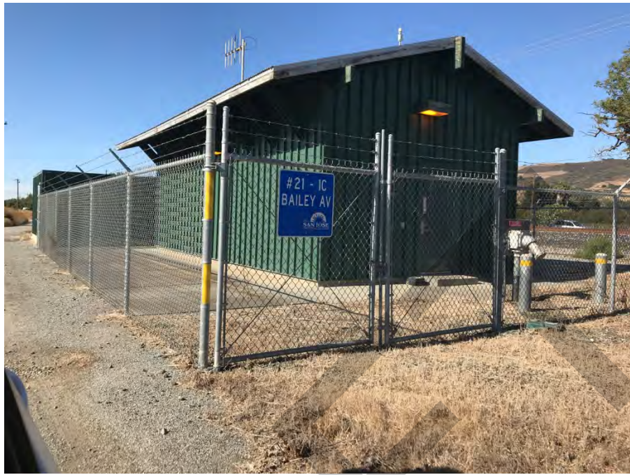
South side of municipal pump house #21-1C and Southeast Perimeter Road
