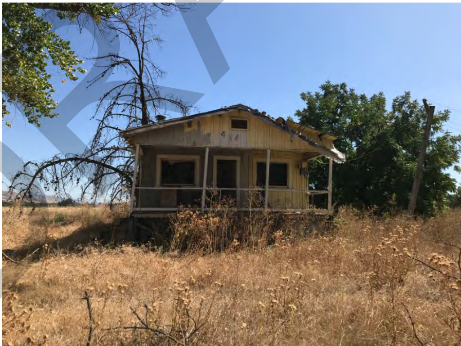
Front of single-family home in Blanchard Residential Area; to be demolished.
