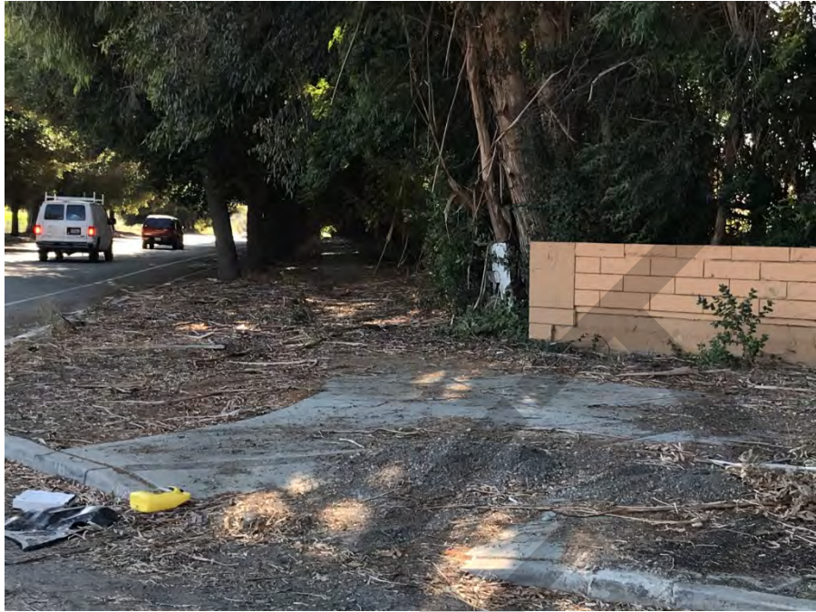
Sidewalks along north side of Bailey Avenue to the west of the turnout.
