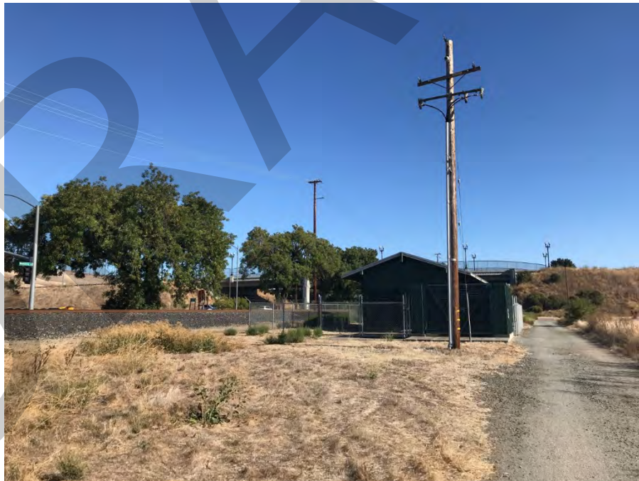
North side of municipal pump house #23-1A and Southeast Perimeter Road
