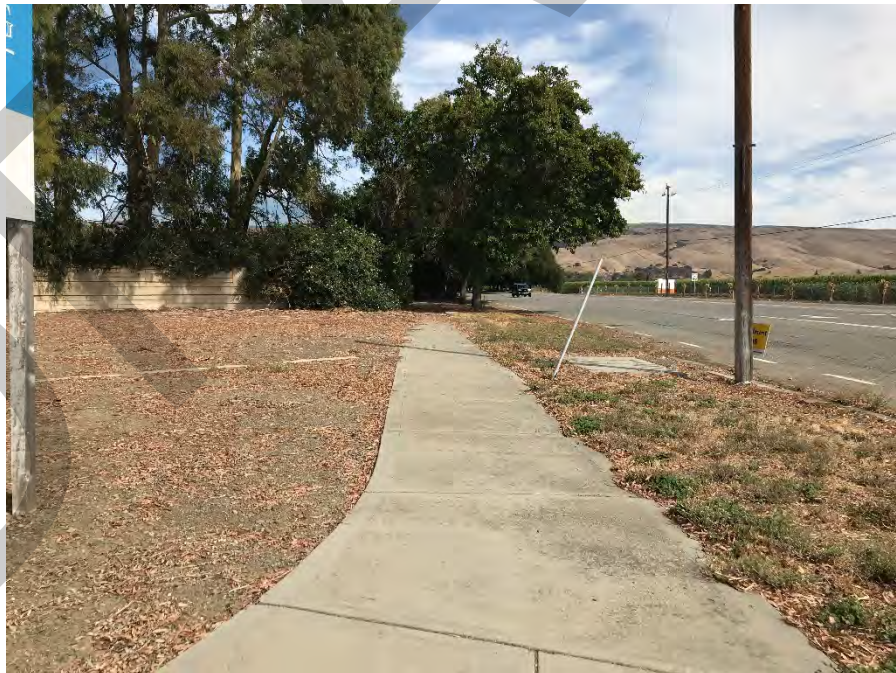
Sidewalk along north side of Bailey Ave. to east of intersection of Santa Teresa Boulevard and Bailey Avenue.
