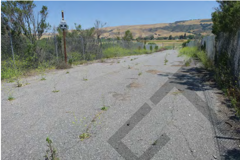
Entrance to Calpine Road from Santa Teresa Boulevard on the western edge of parcel 708-28-002, showing initial stretch of asphalt to gate, and 6' tall chain link fence with 1' of reflexed barbed wire on top.
