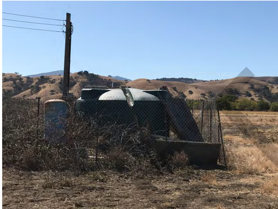
Western view of well, one large green tank and one small blue tank near the center of the Fisher Flats western parcel 708-25-004.
