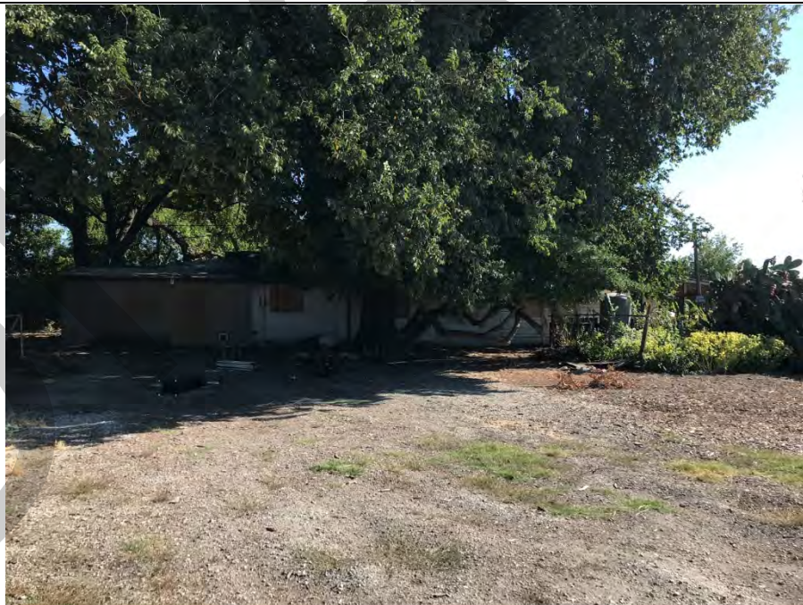
Southern portion of the Emado Compound. North side of western single-family residence with overhang on western side and addition on eastern side. Well and gray tank in front of residence. Debris on ground around the home.
