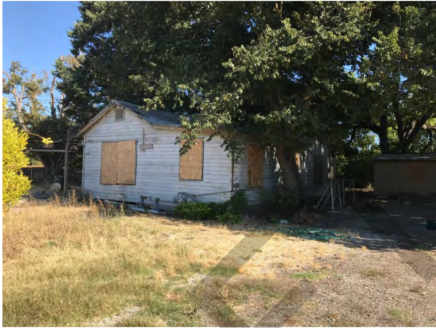
Southern portion of the Emado Compound. North and west side of eastern single-family residence.
