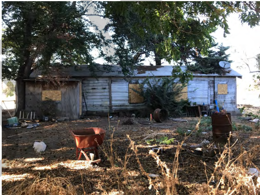
Southern portion of the Emado Compound. Southern side of eastern single-family residence with debris scattered to the south.
