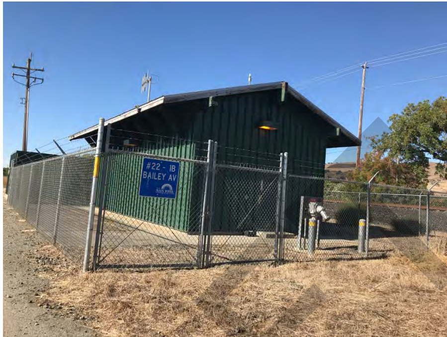
South side of municipal pump house #22-1B and Southeast Perimeter Road
