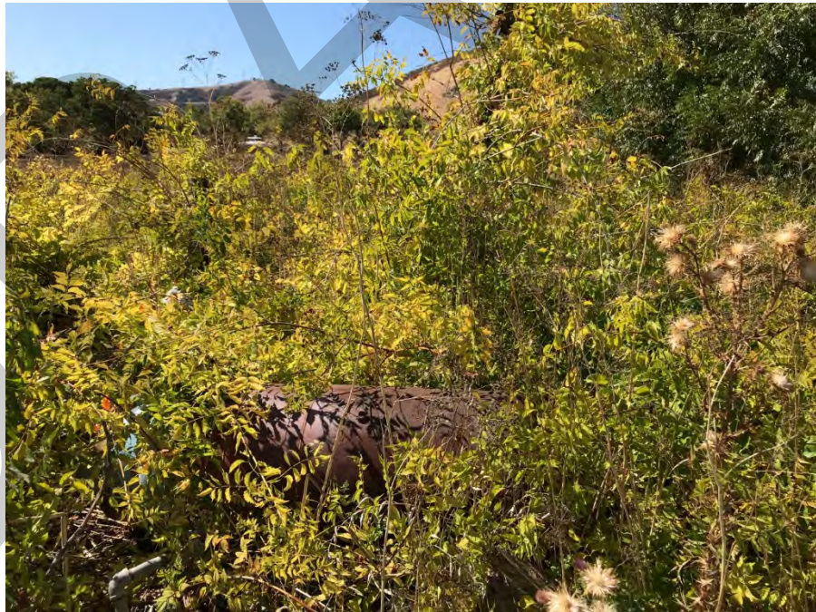
Well in overgrown vegetation behind single-family home in Blanchard Residential Area with rusted tank laying on its side, possibly inactive.
