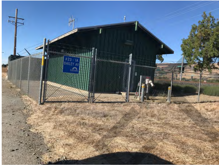
South side of municipal pump house #23-1A and Southeast Perimeter Road
