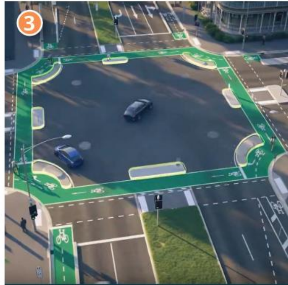
Protected intersections to reduce the speed of turning traffic and conflict points between drivers and bicyclists
