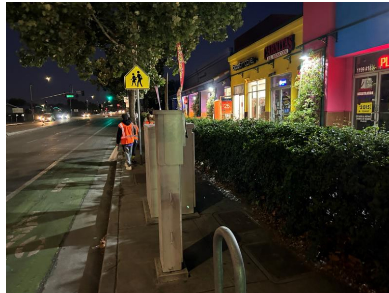
Figure: Sidewalk too narrow for pedestrians
