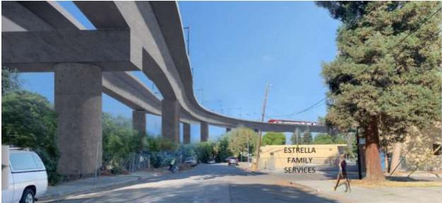
Figure 3 – Four-Track Viaduct Rendering
