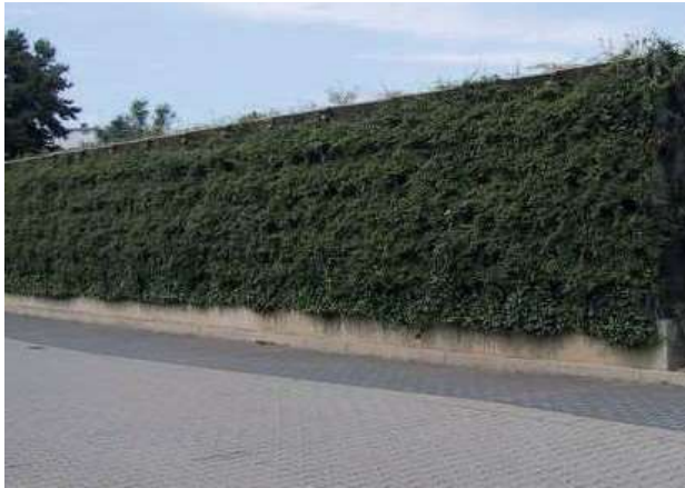
Figure 10 – Sample noise wall mitigation
