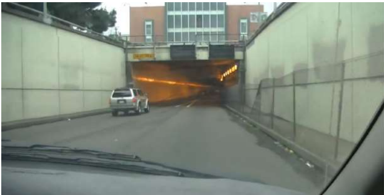
Figure 6 – Posey Street Tube, Oakland to Alameda
